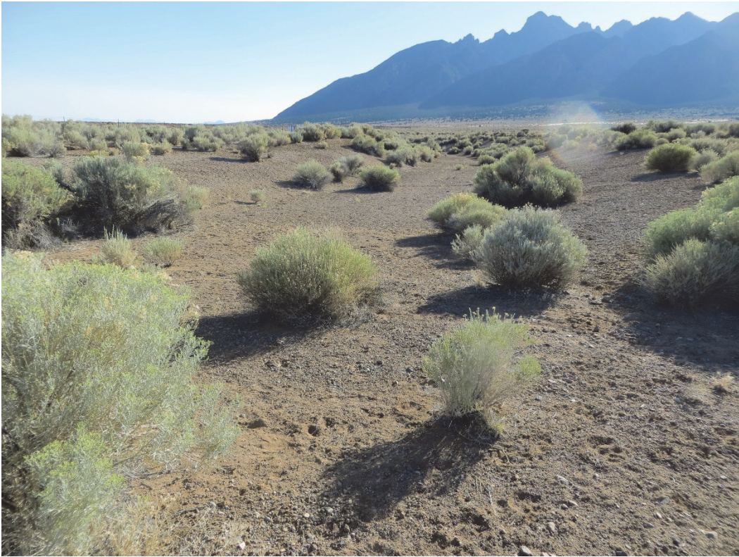
Photograph 5. UC-1 West Stormwater Diversion Channel (view from site access road, looking southwest)
