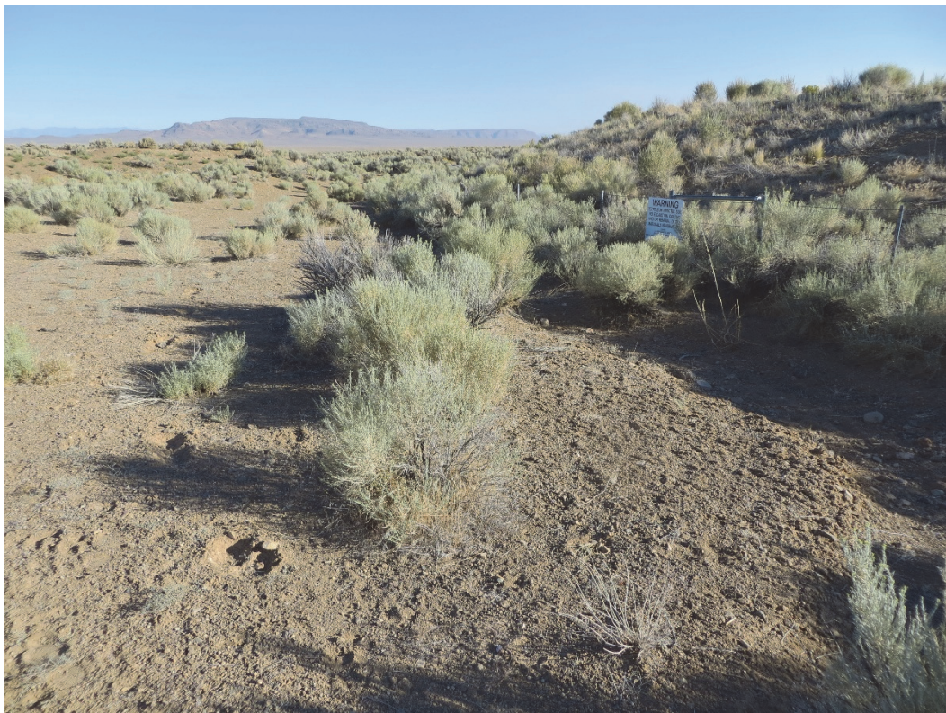
Photograph 4. UC-1 East Stormwater Diversion Channel (view from site access road, looking south)
