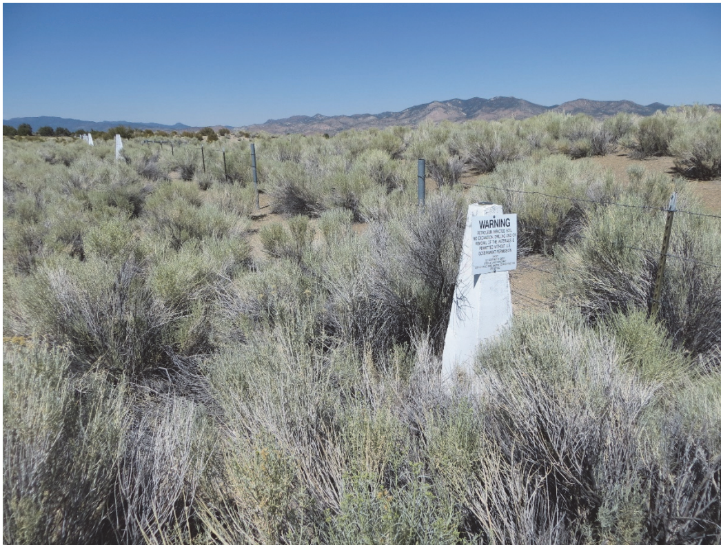
Photograph 11. UC-4 Mud Pit C (view of entrance to fenced area with missing gate, looking northeast)
