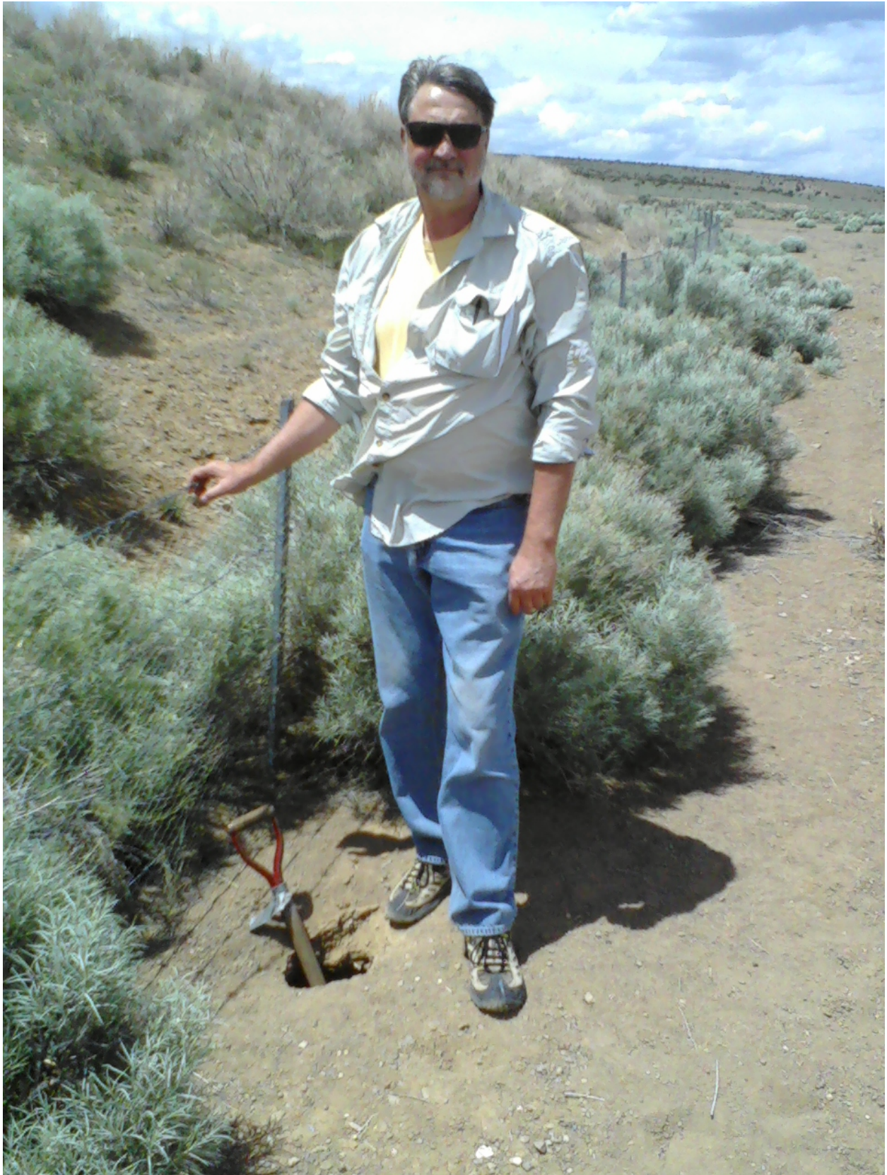
Photograph 15. UC-1, Possible piping structure near east toe of cap
