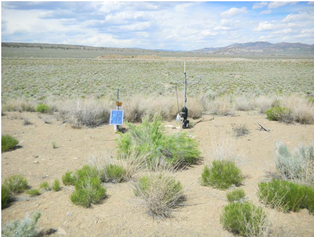
Photograph 3. UC-1, View from south edge looking north
