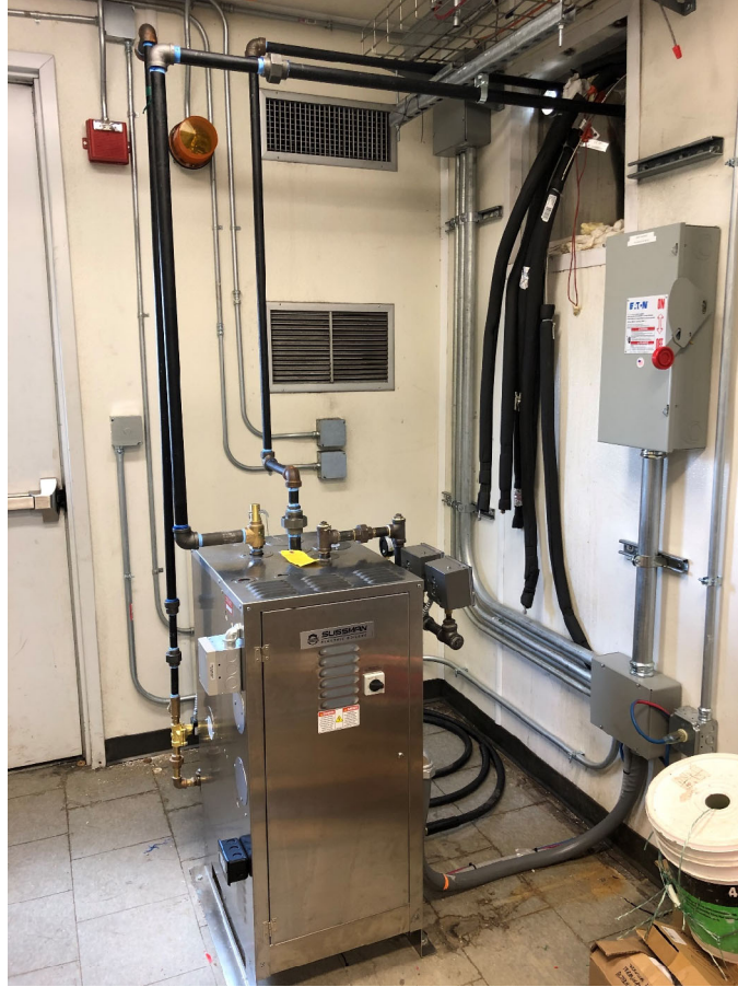
Figure 7-17. An electrical steam generator installed inside the trailer.
