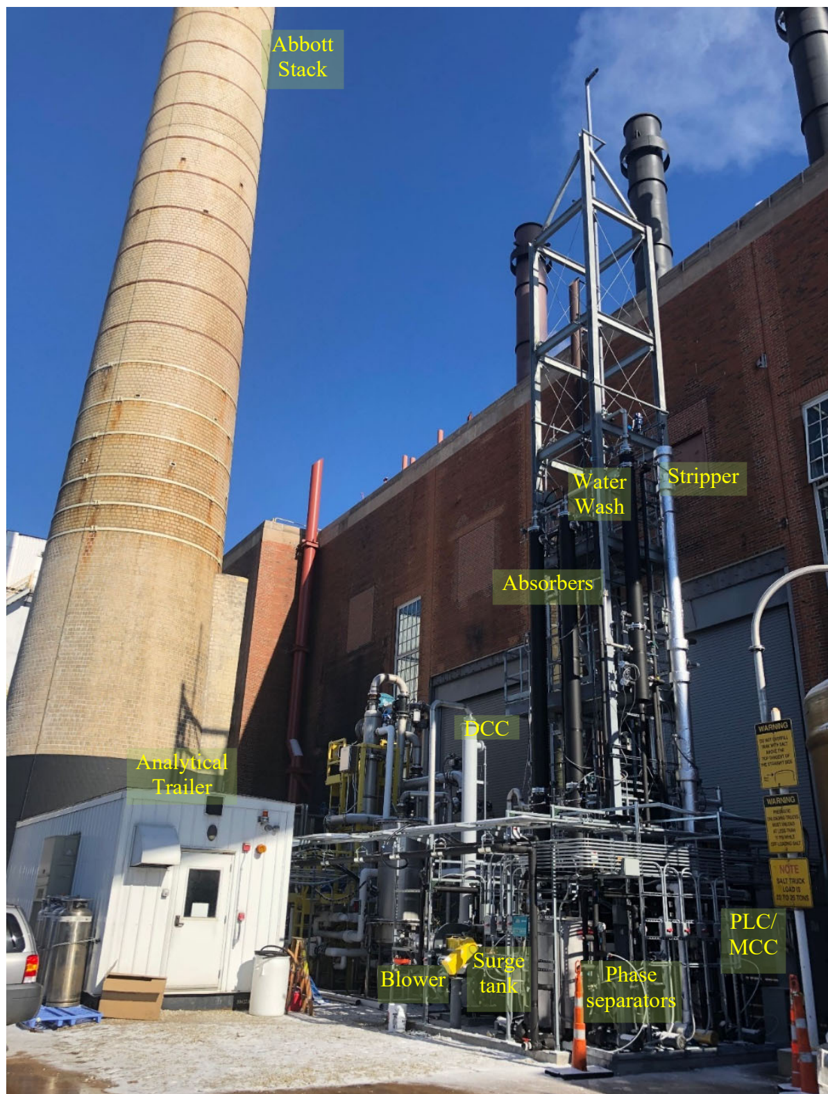
Figure 7-9 Biphasic skid installed at Abbott Power Plant.
