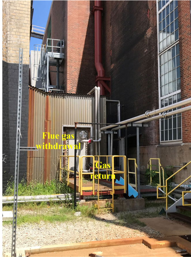
Figure 7-10. Flue gas piping from and returning to Abbott stack.
