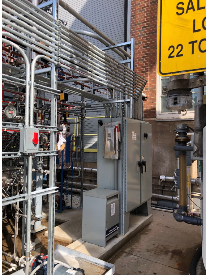
Figure 7-14. PLC/MCC panels for the bench-scale BiCAP skid.
