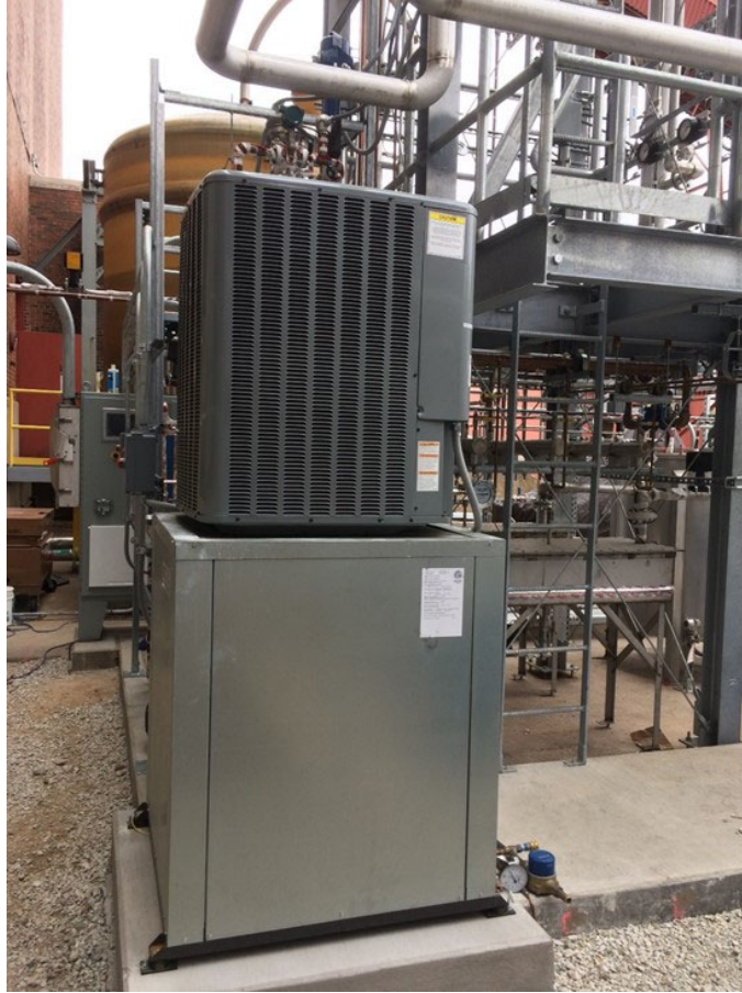
Figure 7-13. Chiller installed outdoor for providing cooling water for the BiCAP skid.
