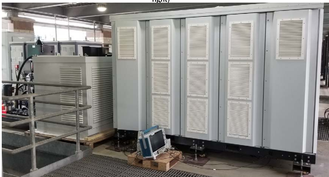
Figure I.1.1.7 400kW XFC Setup Front View (SST, Charger Power Cabinet, Dispenser, and DCE from left to right)
