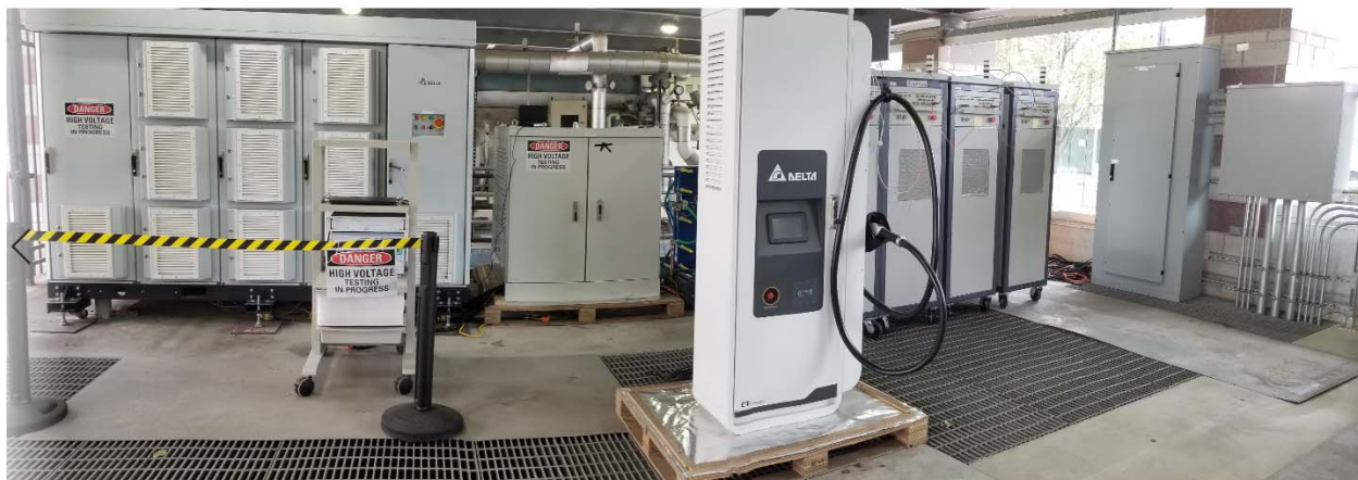
Figure I.1.1.7 400kW XFC Setup Front View (SST, Charger Power Cabinet, Dispenser, and DCE from left to right)
