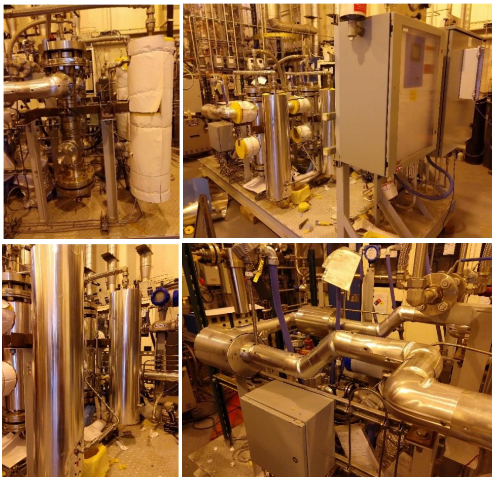
Figure 3. Reactors and piping on the skid were first insulated with fiberglass (top left) and then sheathed in aluminum.
