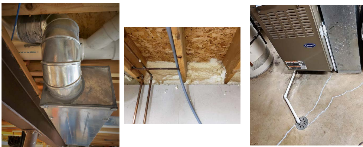
Figure 2. Treatment measures included duct sealing (left), air sealing and insulating rim band joists (middle), and air sealing crawl space and basement slabs (right).
