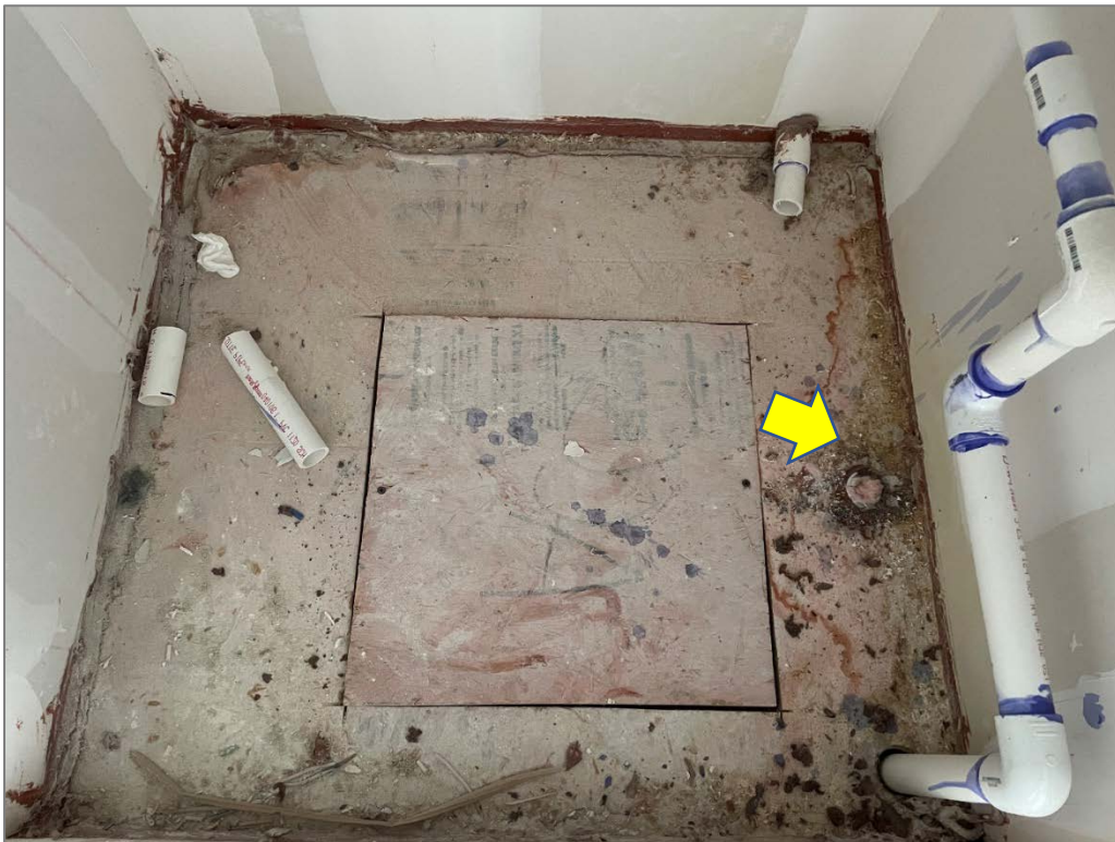
Figure 8. Unsealed condensate access (note relocated drain hole filled with batt insulation)
