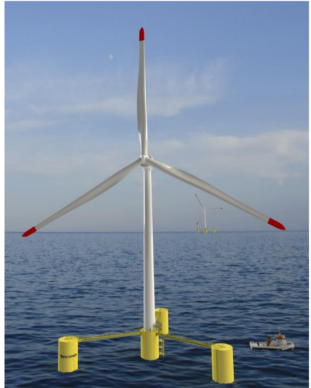
Figure 11 The New England Aqua Ventus I Project will Demonstrate the VoltturnUS Concrete Floating Hull
