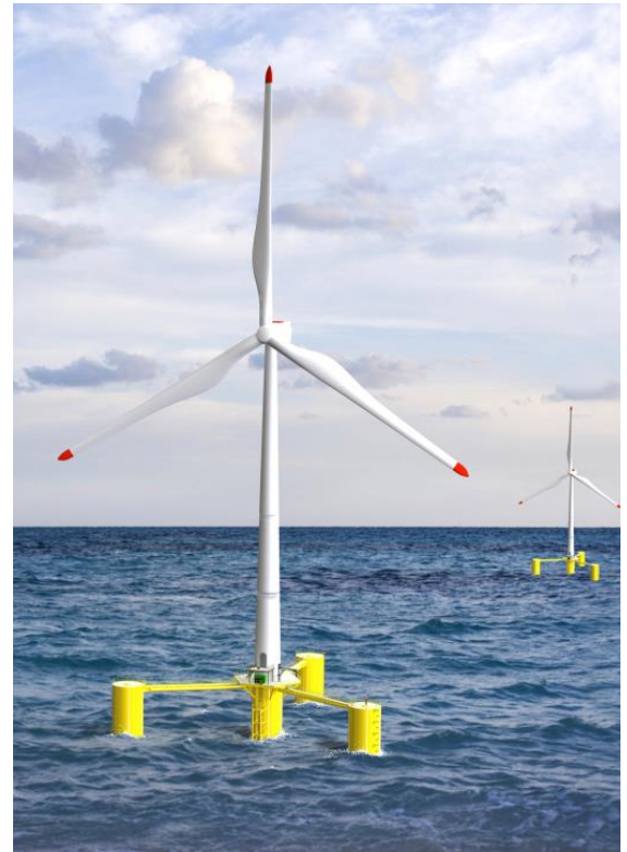
Figure 2 In BP 1 the Aqua Ventus I Project Consisted of Two 6MW Wind Turbines Supported atop VoltornUS Concrete Floating Hulls
