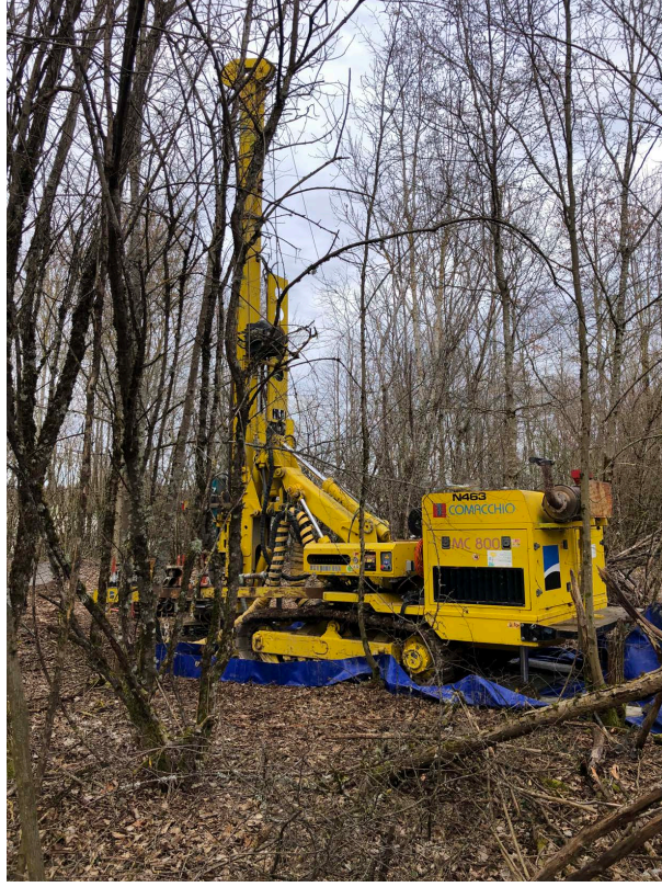
FIG. 8. Photo of the ongoing drilling of a core at the proposed FPF location to assess the geological conditions.
