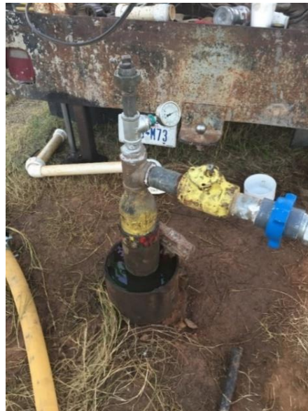
Figure 6-7: Wellhead assembly, consisting of an analog pressure gauge, connections to the injection well casing, and the shutoff valve (the yellow valve on the horizontal segment of the wellhead assembly), which was connected to the 300-ft long surface pipe. The In-Situ TM bottomhole digital pressure and salinity transducer was suspended by a 177-ft long rope hanging from the end cap above the analog gauge.
