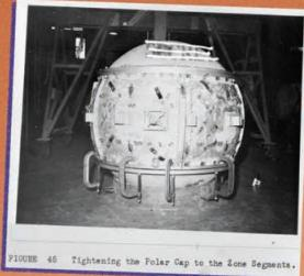
FIGURE 45 Tightening the Polar Cap to the Zone Segments.
