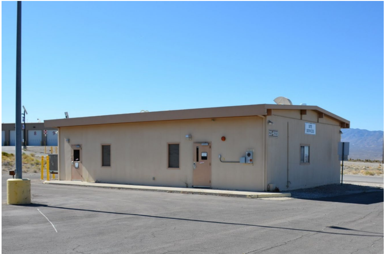
Figure 10. Building 23-620 north and east elevations, facing southeast (22110_3932, DRI 2022).
