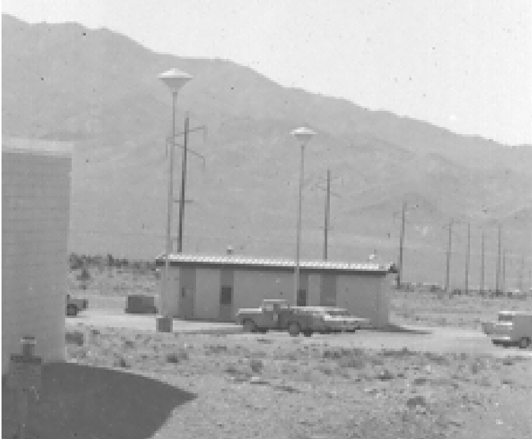
Figure 5. Building 23-620, north elevation, March 4, 1971, facing south (best copy available) (REEC0 3316-14).
