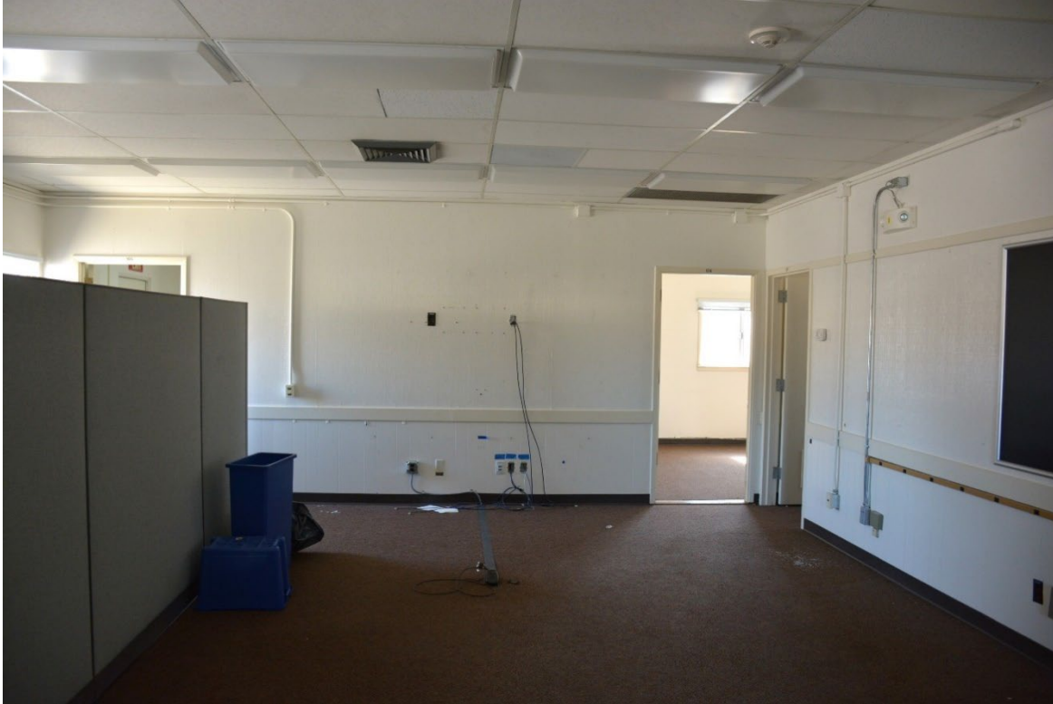
Figure 12. Interior of Building 23-620, main office area, facing east (22110_3945, DRI 2022).
