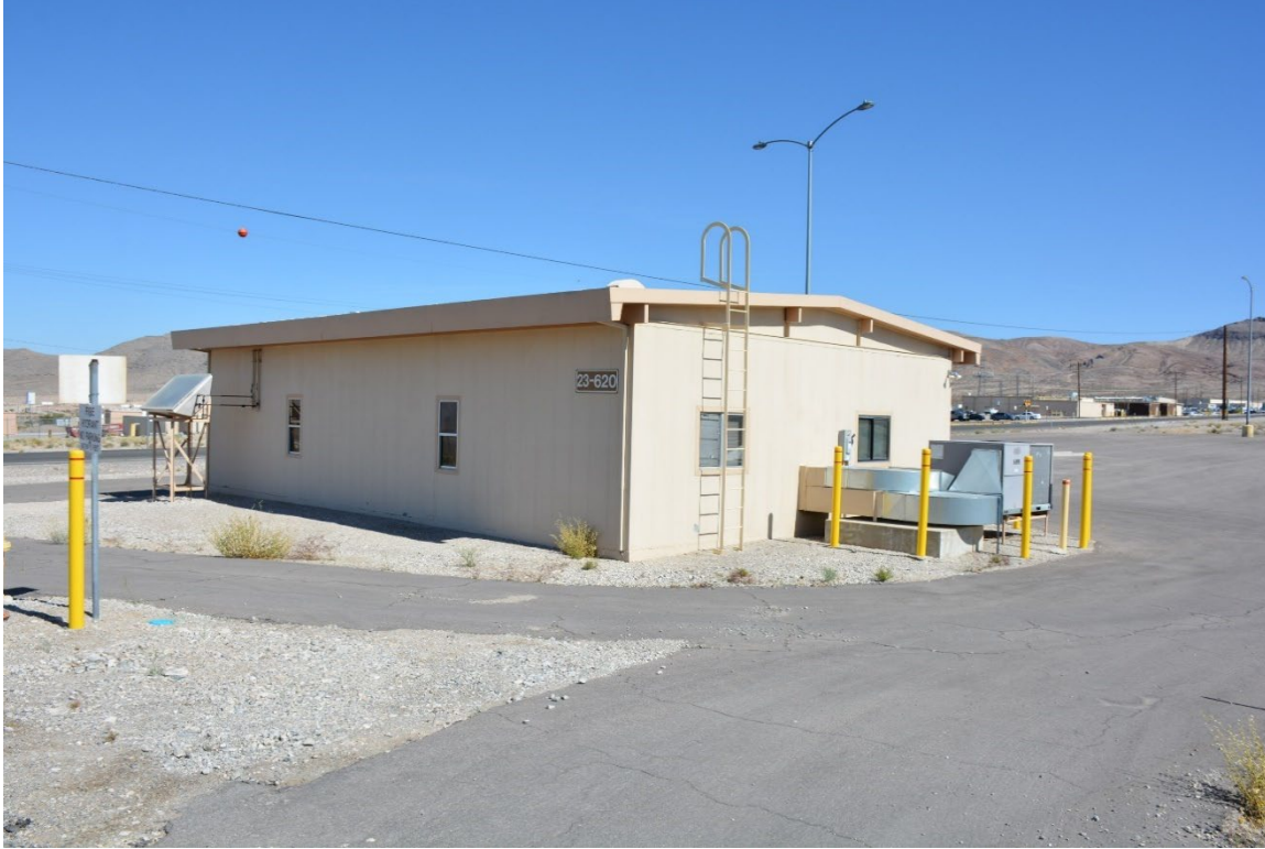
Figure 11. Building 23-620, south and east elevations, facing northwest (22110_3938, DRI 2022).
