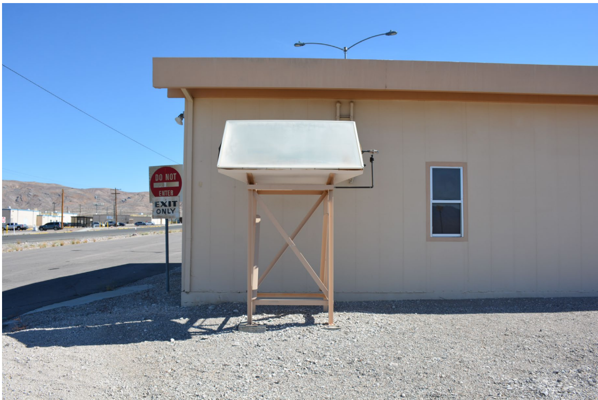
Photograph 10. Close-up of solar water heater (22110_3937). Elevation: South Direction facing: North Photographer: Brannan Date: 05/24/2022
