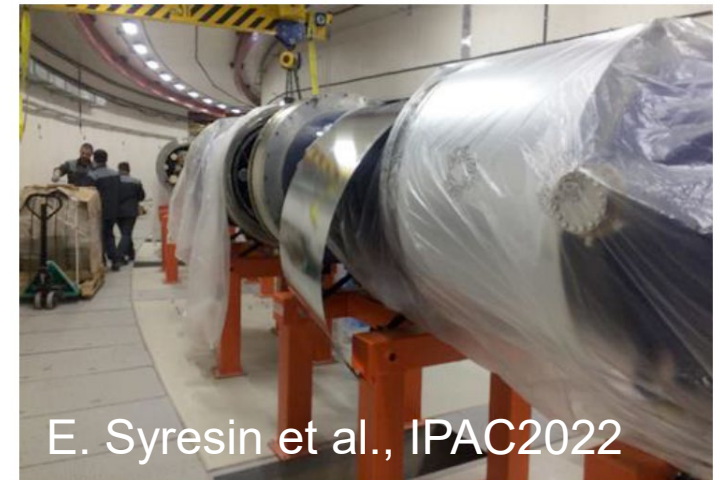
Figure 5: Installation of magnets in NICA tunnel.
