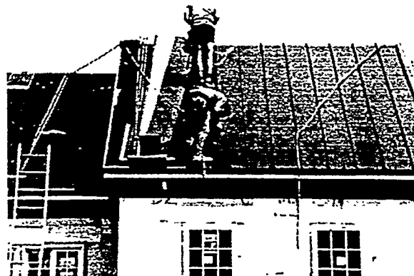
Figure 16 Clips Installed to Hold the Metal Panel
