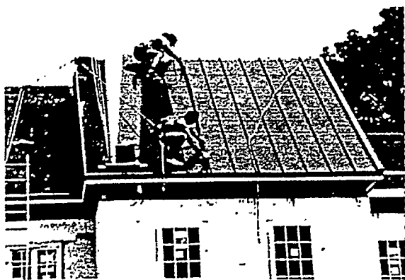
Figure 17 Batten Placed Over the Standing Seam
