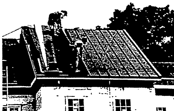
Figure 14 Placement of Metal Roofing Panel
