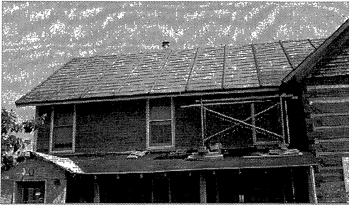
Figure 5. The horizontal batten seam BIPV system as installed on the Beaver Island Blue Bird Bed and Breakfast.
