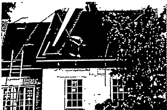
Figure 15 Metal Roofing Panel Slid Into Place
