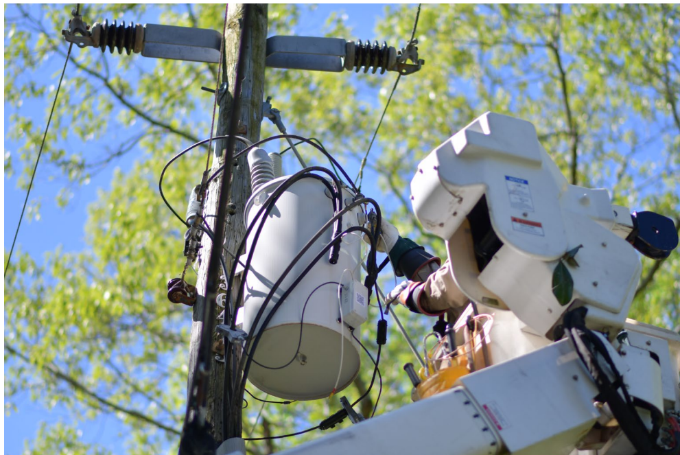
Figure 7 Sensor installation
