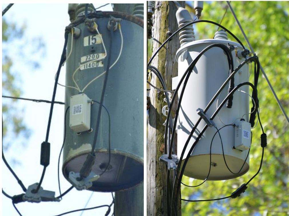
Figure 5: Transformer monitors in the field
