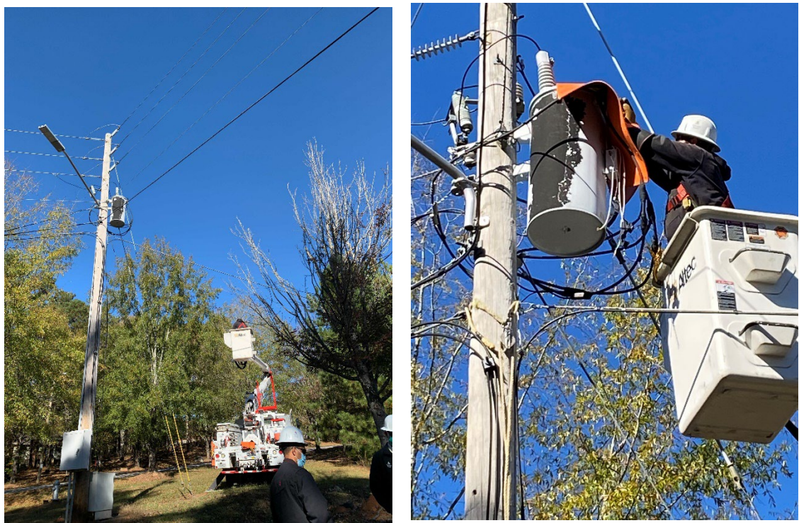
Figure 3: Sample #1 being installed on a “live” transformer
