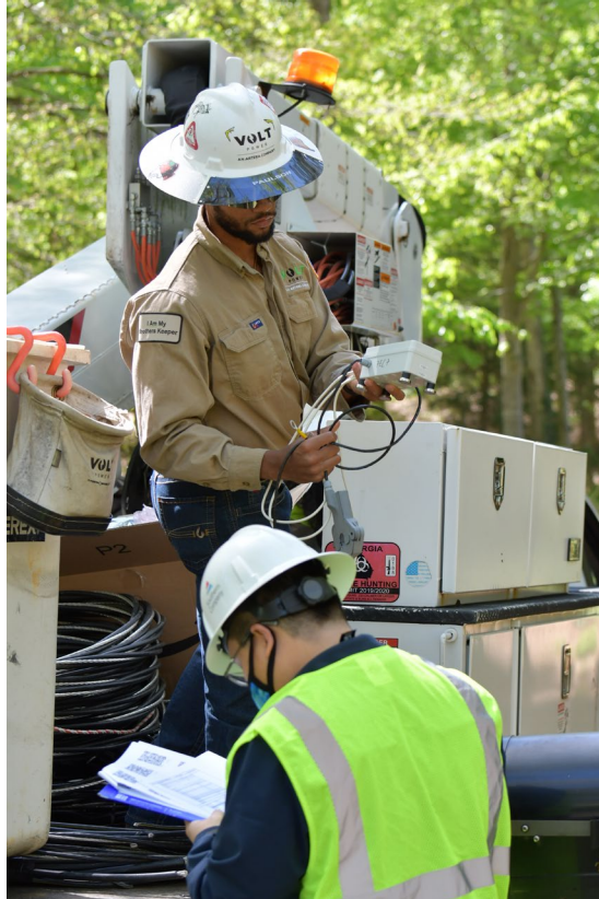
Figure 6 Utility lineman handling and installing the sensor in the field
