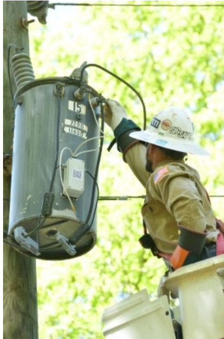
Figure 4: A transformer monitor being installed in the field
