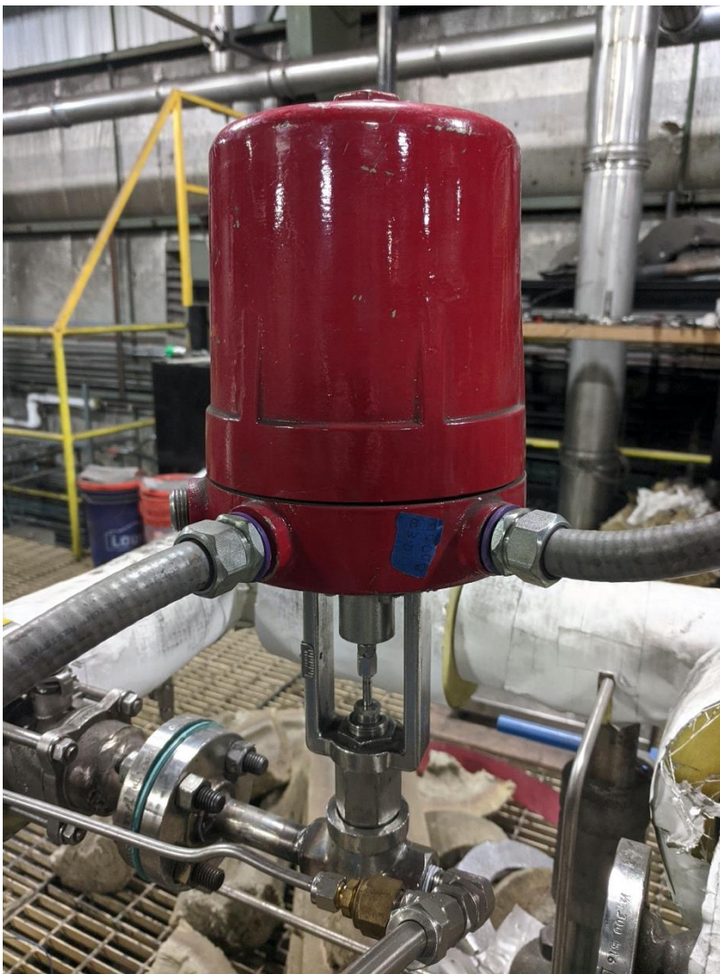
Figure 63. Electronically actuated control valve (Badger valve)
