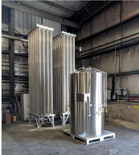
Figure 35. Placement of CO 2 microbulk tank at the University of Utah’s Industrial Combustion and Gasification Research Facility
