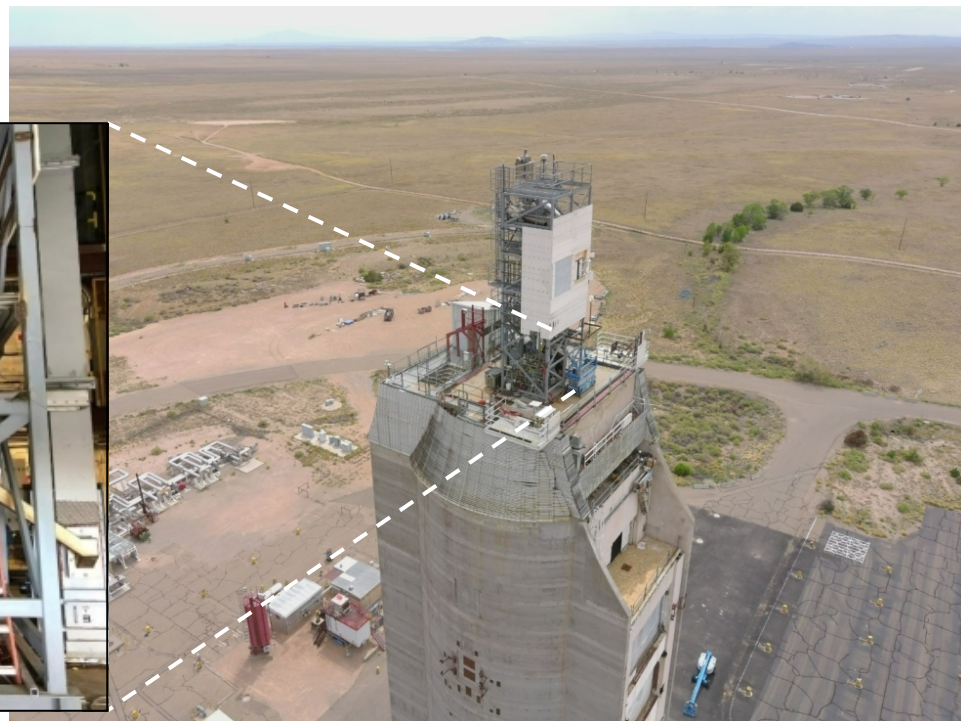
On-sun testing of integrated system with falling particle receiver
