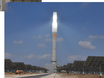
Gemasolar, molten salt, 19 MW e , Spain, 2011
