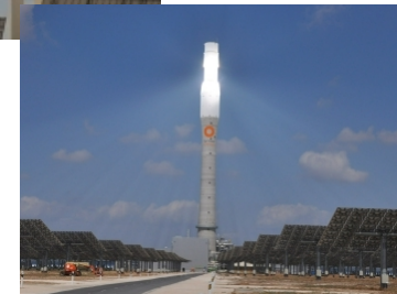
Gemasolar, molten salt, 19 MW e , Spain, 2011
