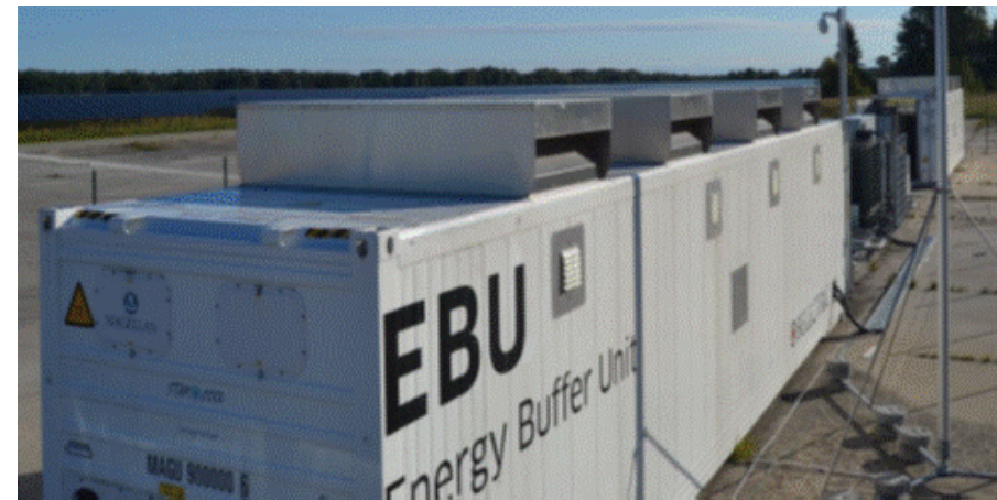
1.3MW/1.9 MWh advanced lead acid battery system providing support for a 68MW solar farm in Alt Daber, Germany (Source: BAE Batteries, 2018)
