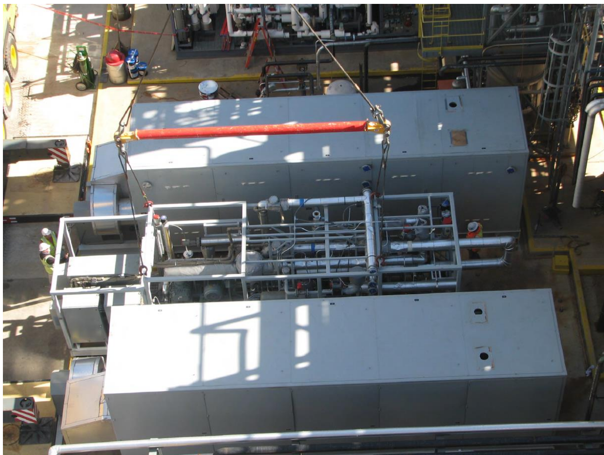
Figure 36. Installation of TDA Pilot unit on-site at NCCC
