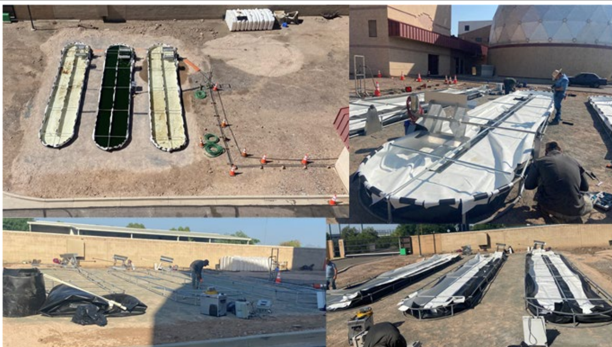
Figure 7.1. Installation of the three 25-m 2 raceways at the City of Mesa Northwest Water Reclamation Plant.
