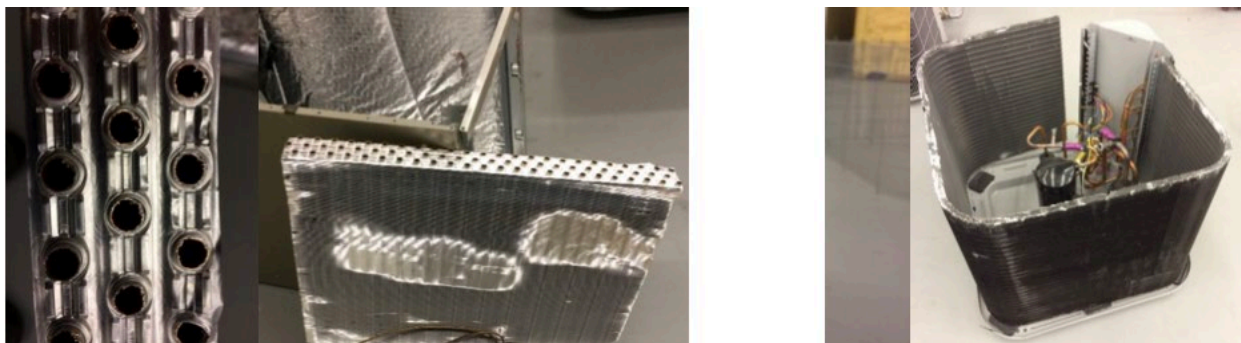
Figure 5: Baseline Heat Exchangers for a 2.5-ton heat pump; a) Indoor b) Outdoor
