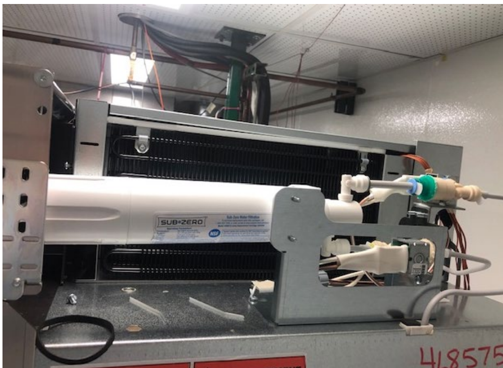
Figure 100: Wire on Tube Baseline Heat Exchanger in Sub-Zero System Assembly
