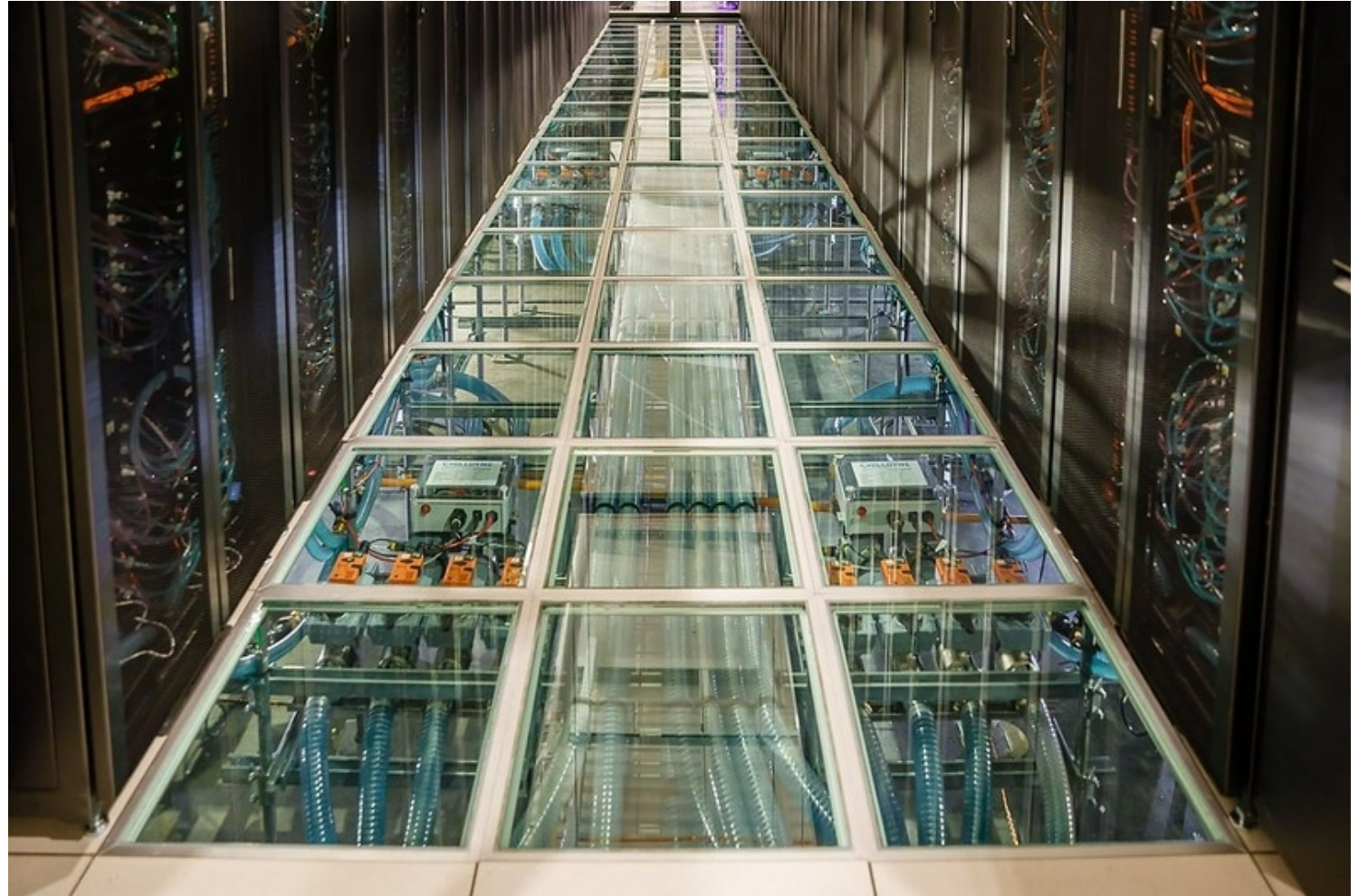
Water-cooled server racks in Sandia's High Performance Computing data center. (Photo by Bret Latter)
