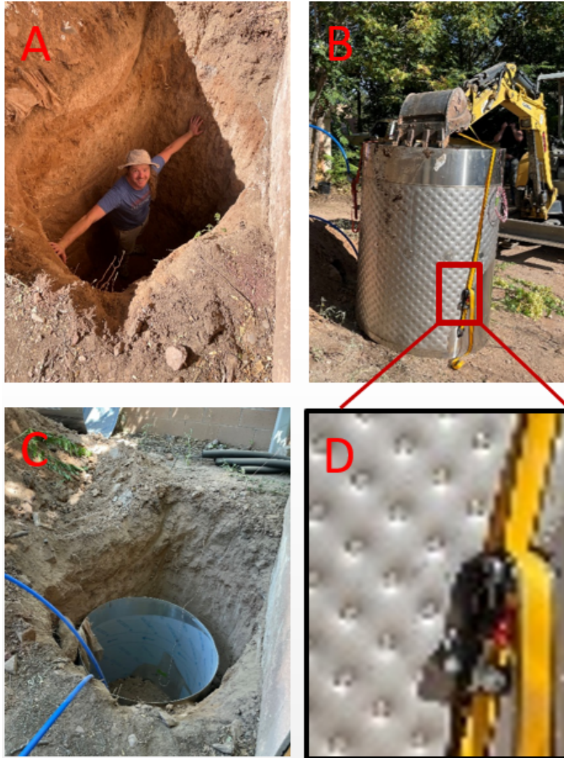
Figure 1-2. 2A. Patrick Johnson inside a ground cavity that was excavated for the dimpled heat exchanger. 2B. Full-scale, fully-passive, dimpled heat exchanger. 2C. Heat exchanger lowered into the soil. 2D. Surface zoom showing the dimples that provide enhanced heat transfer.
