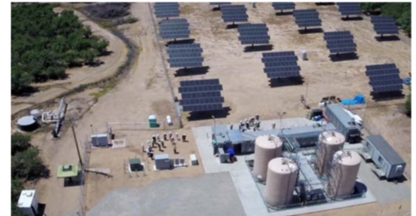
Figure 3. Photograph of EnerVault Corp.'s 250kW/1MWh Fe-Cr RFB in Turlock, California. Electrolyte is held in the four tanks in the lower right [34].
