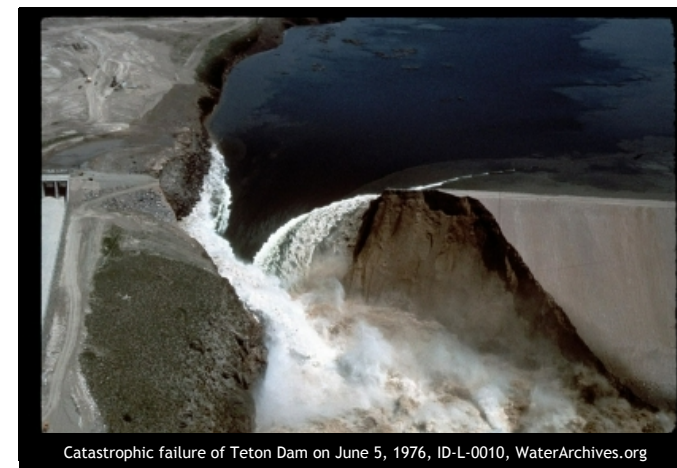
Catastrophic failure of Teton Dam on June 5, 1976, ID-L-0010, WaterArchives.org
