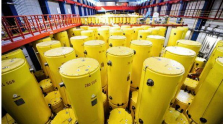
Figure 5: Some facilities have tightly packed casks, and access to seals at the top of casks is achieved via crane or bridge. Image from [8].
