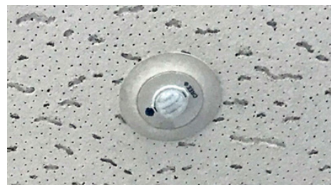
Lunch room LED fixtures after retrofit, a significant energy savings and improvement in lighting quality.
