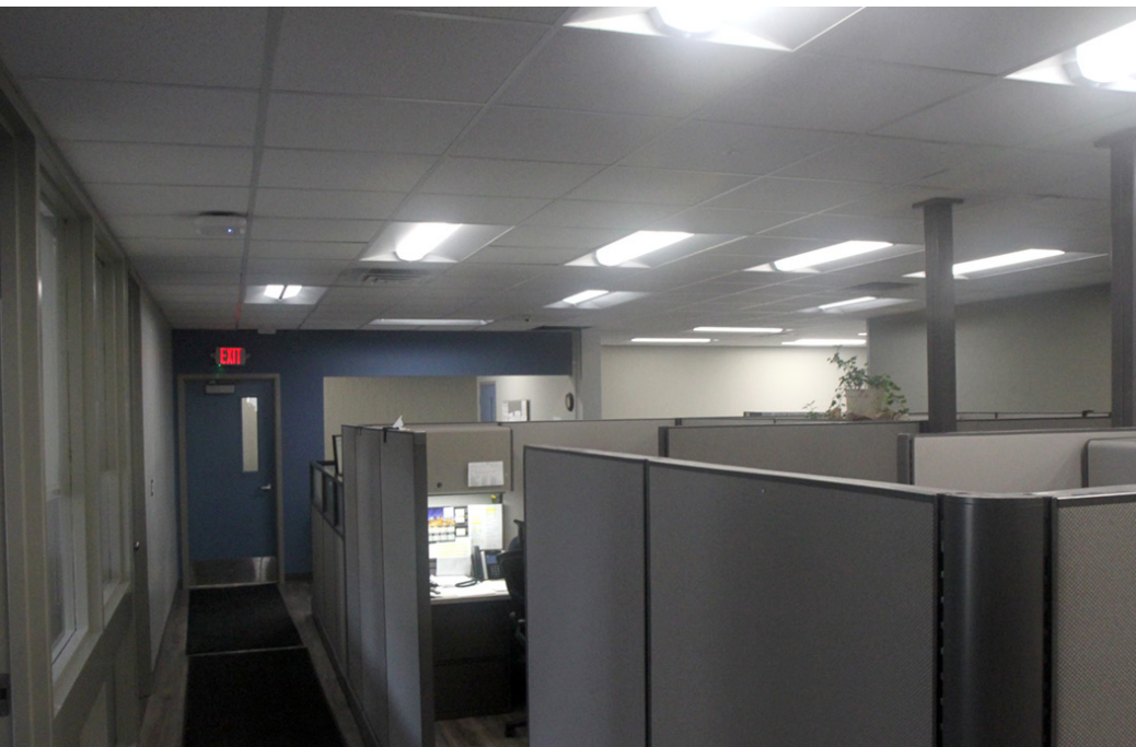
(Above) LED troffers above the open office area cubicles; (Right) Existing BAS controllers.
