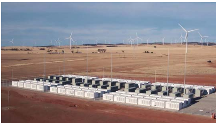
Tesla 100 MW / 129 MWh ESS Australia - Grid stability
