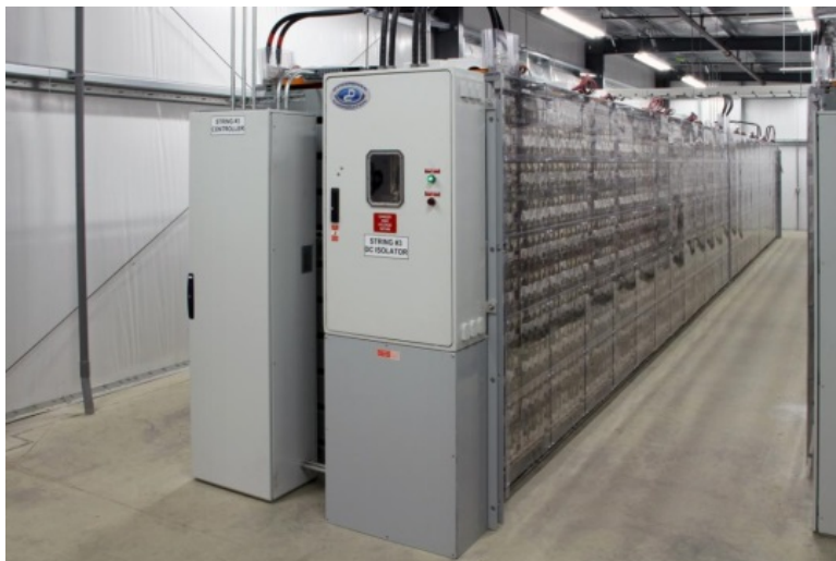
3 MW/3 MWh advanced lead acid battery system for utility applications (Source: EastPenn, East Lyons, PA)
