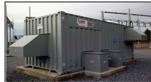
FIAMM 222-kWh System Duke Energy Rankin Substation
