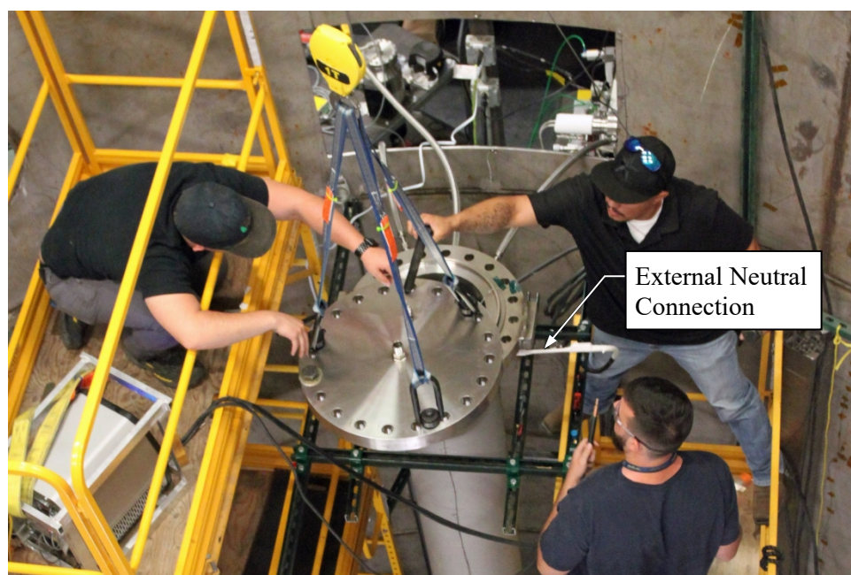
Figure 3-2 Installation of top flange.
