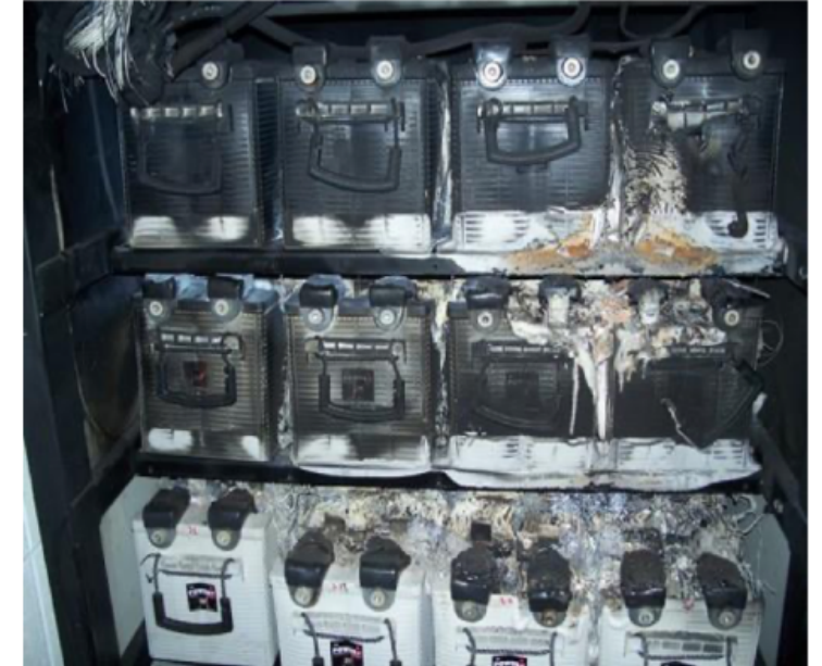
Fire damage from VRLA thermal runaway
