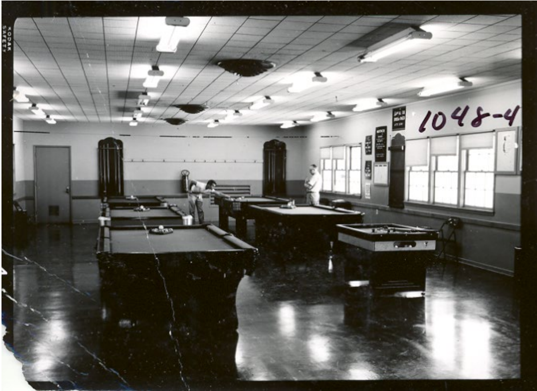
Billiards tables in Recreation Hall. Elevation: N/A Direction facing: N/A Photographer: REECo Date: 8/1/1961
