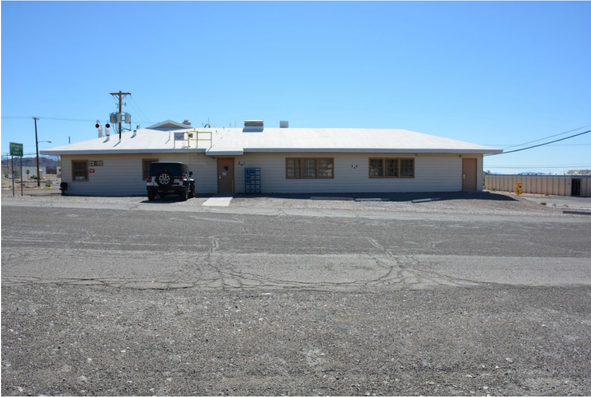
PHOTOGRAPH 5. NORTH ELEVATION, FACING SOUTH (2237_3587, DRI 2022).
