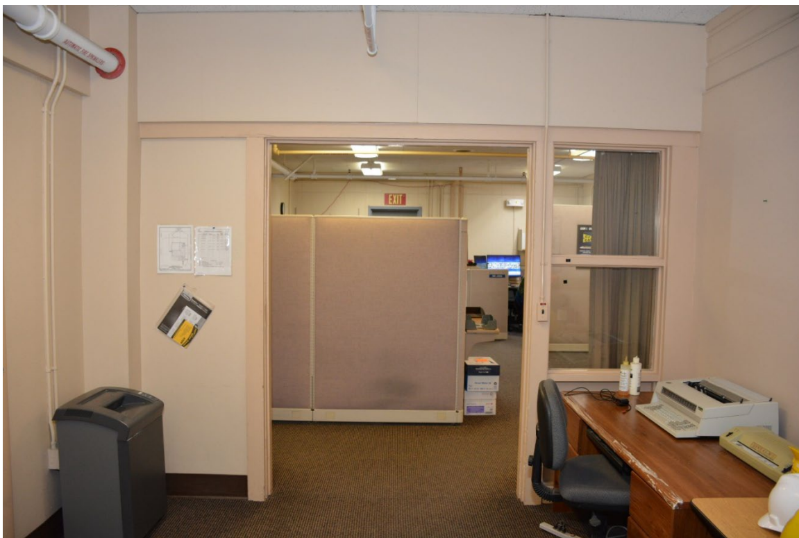
PHOTOGRAPH 14. ROOM 3 (FORMER PORCH), FACING NORTH (2237_3548, DRI 2022).
