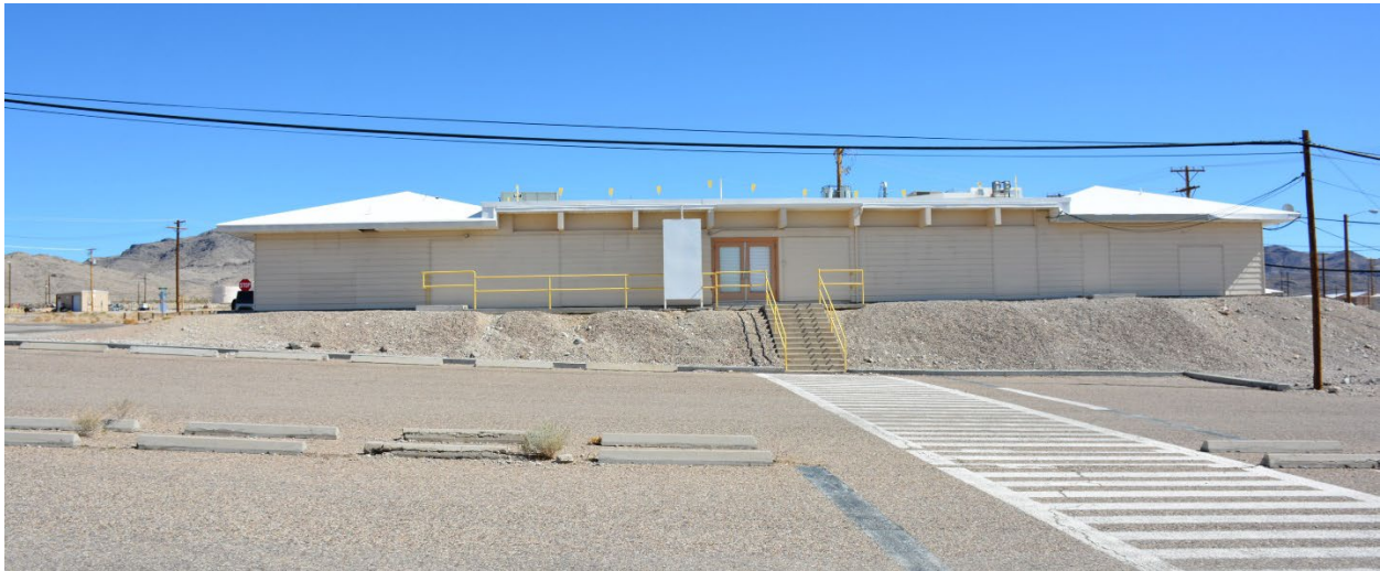
Figure 15. West elevation of Building 23-113, facing east (223723_3595, DRI 2022).
