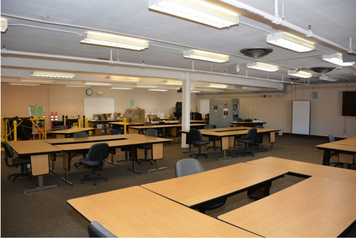
Figure 16. Classroom with exposed rafter beams (223723_3541, DRI 2022).
