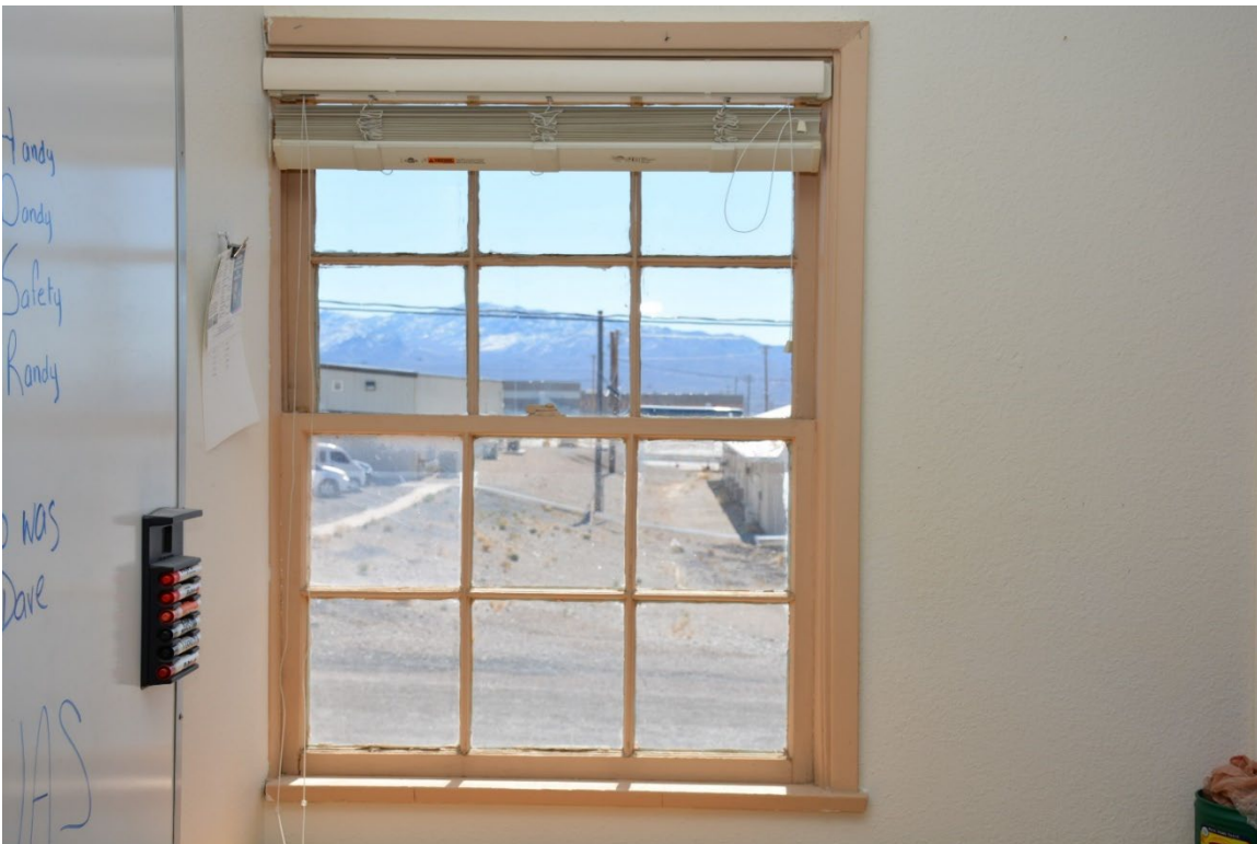
PHOTOGRAPH 20. WINDOW DETAIL IN ROOM 23, FACING SOUTH (2237_3570, DRI 2022).
