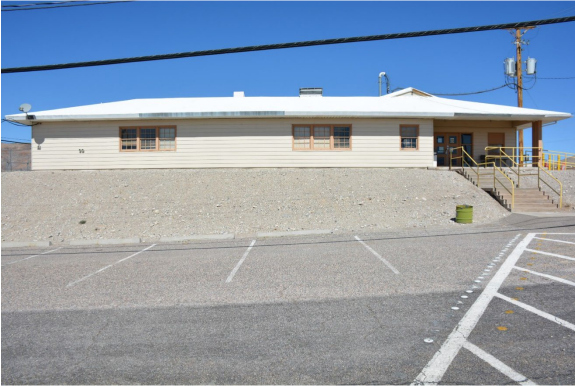
PHOTOGRAPH 1. SOUTH ELEVATION, FACING NORTH (2237_3534, DRI 2022).
