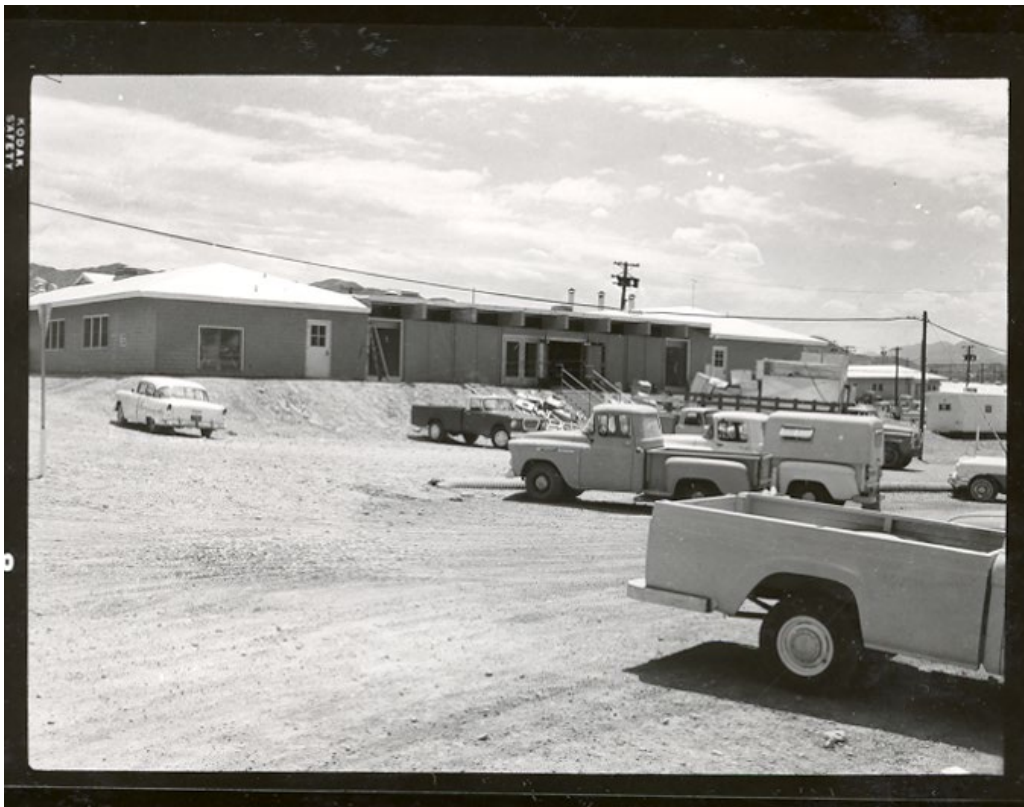
Recreation Hall modifications in 1963 (frame 1673-8).
