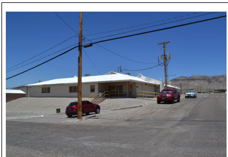
Building 23-113, view northwest (2017).
