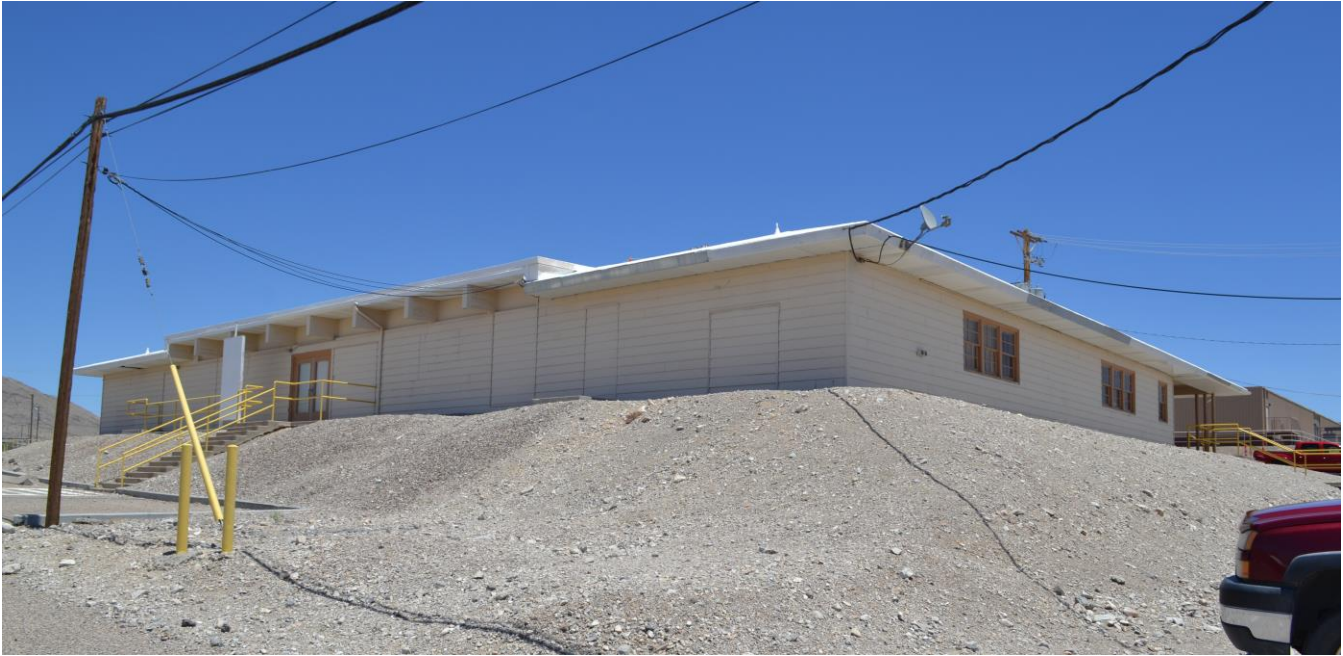
Elevation: South, West Direction facing: Northeast Photographer: Menocal Date: 06/21/2017
