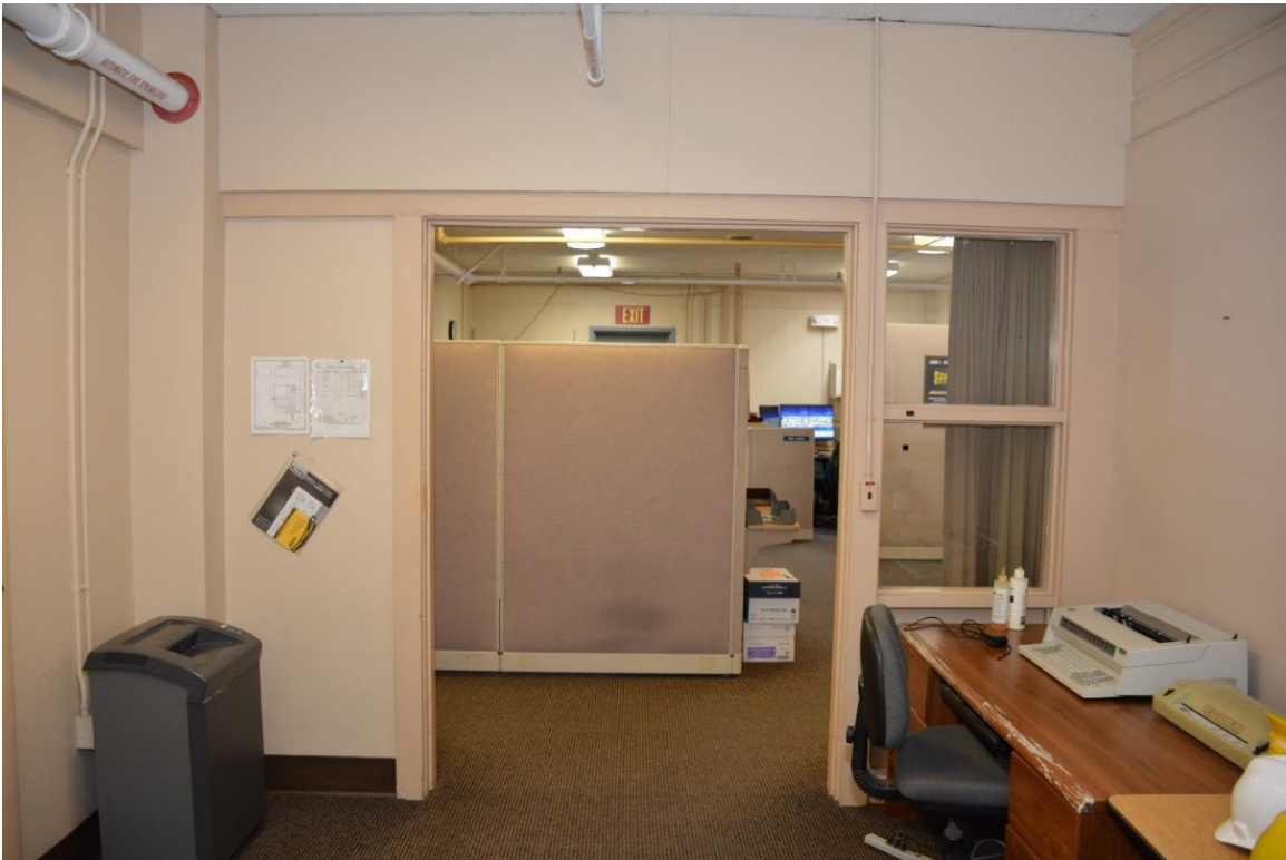
Figure 17. Western entrance of the original porch, now an entrance to a training center/classroom (223723_3548, DRI 2022).
