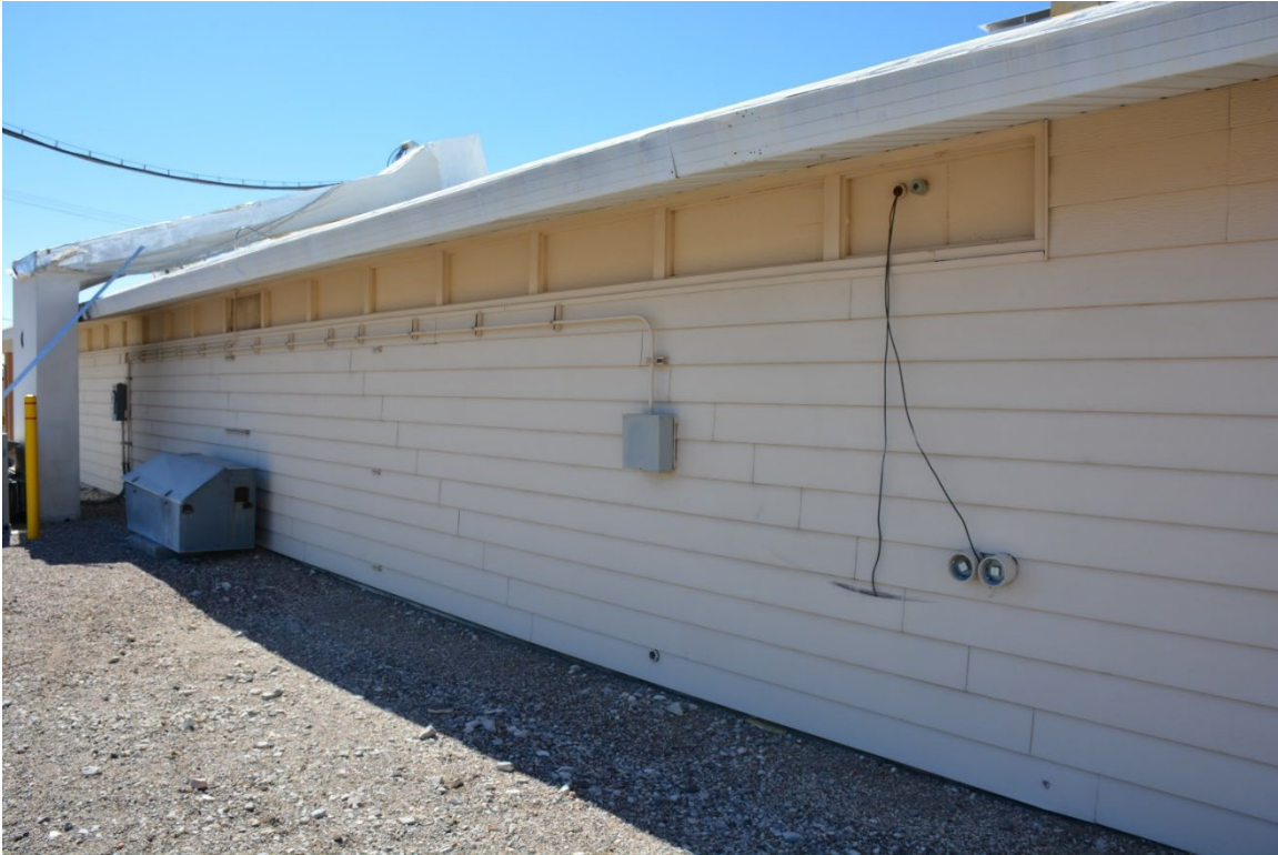
PHOTOGRAPH 3. GYPSUM BOARD COVERED RIBBON WINDOW ON EAST ELEVATION, FACING SOUTHWEST (2237_3583, DRI 2022).
