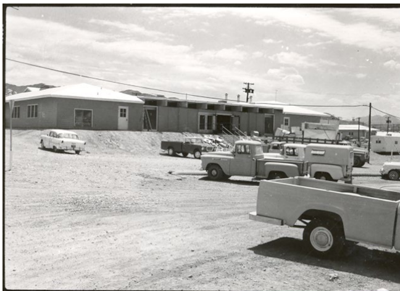
Figure 10. Building 23-113, during modifications, July 31, 1963 (REEC0 1673-8).
