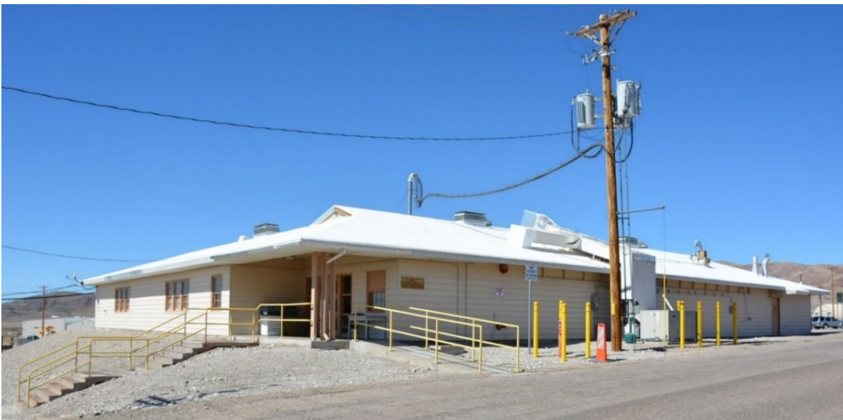
Figure 14. Building 23-113, south and east elevations, showing the main entrance, facing northwest (223723_3579, DRI 2022).
