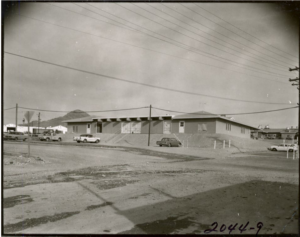
Recreation Hall after modifications were completed.
