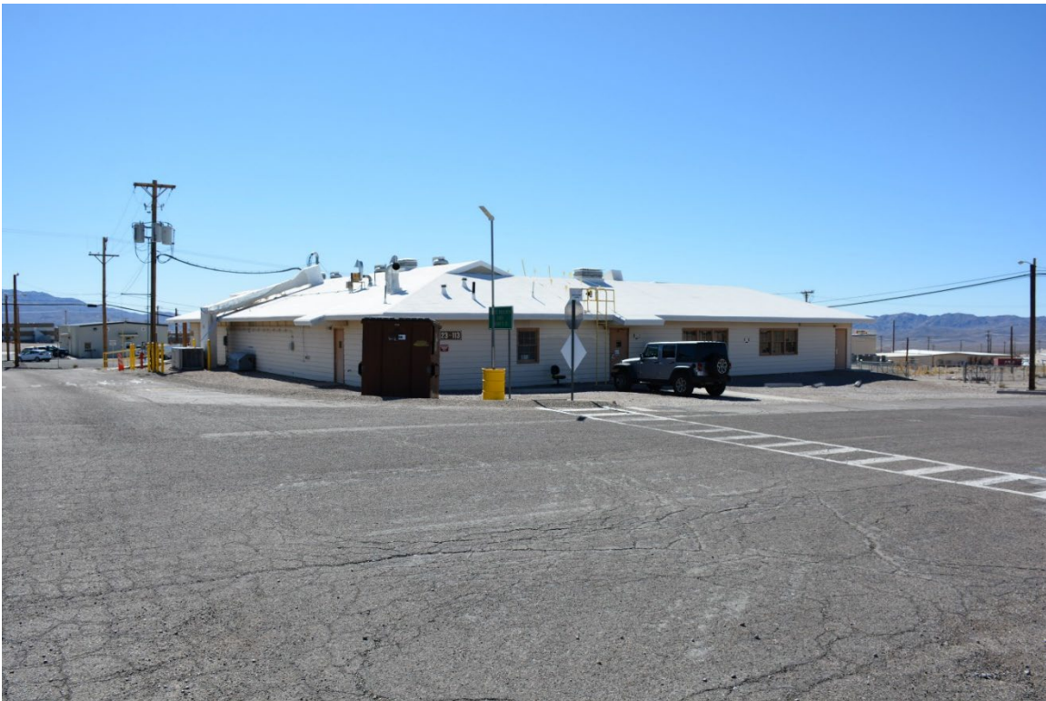
PHOTOGRAPH 4. OBLIQUE VIEW OF EAST AND NORTH ELEVATIONS, FACING SOUTH-SOUTHWEST (2237_3584, DRI 2022).
