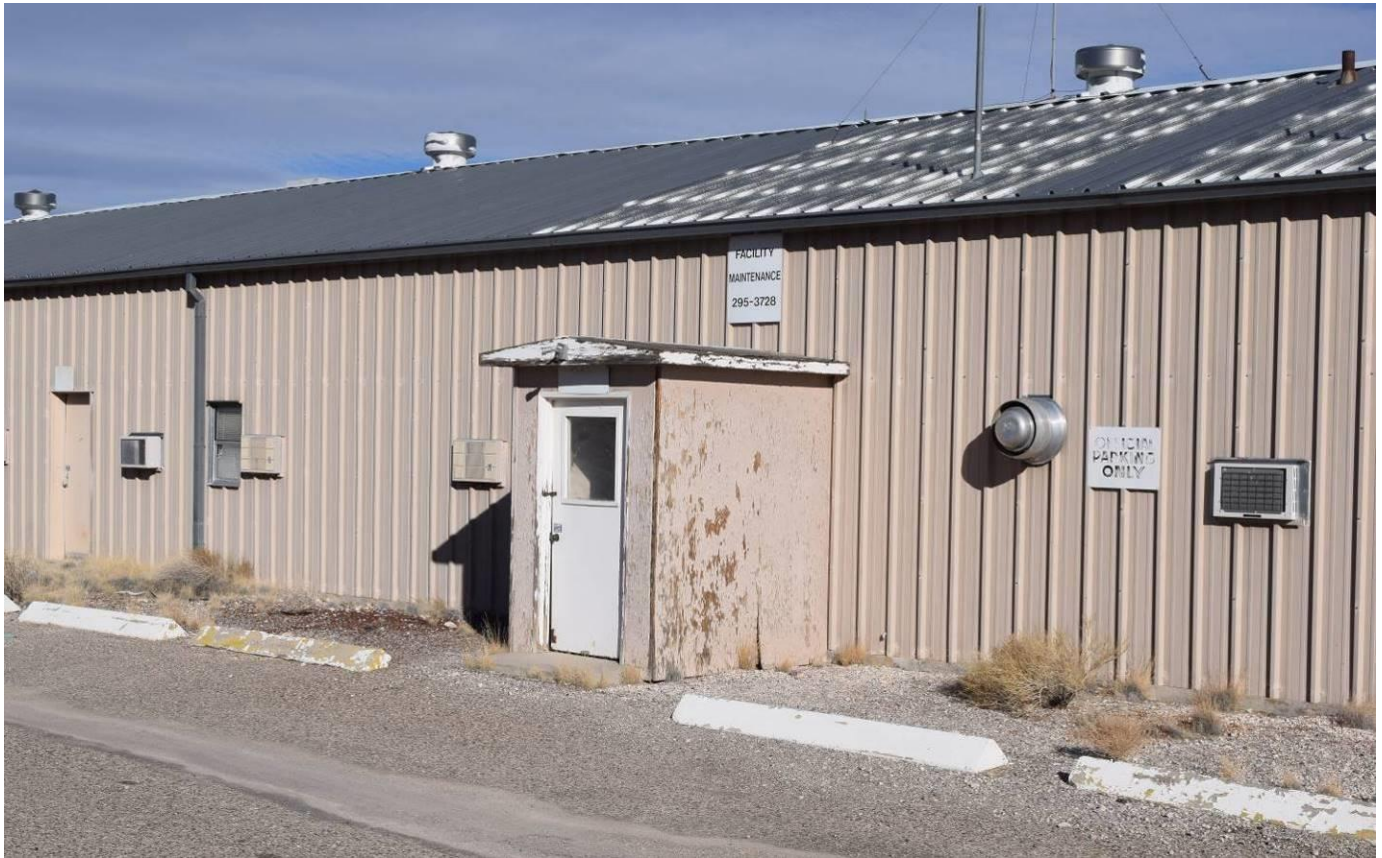
Elevation: West Direction facing: Northeast Photographer: Shaw Date: 1/18/2019 Plywood door enclosure on west side of B17823. Note vents and HVAC units set into walls.
