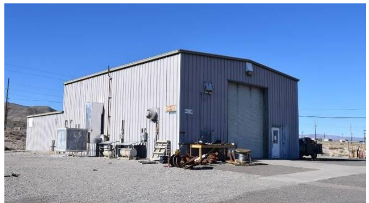
South and east side of Building B17822. View west (2018). Note roll up and pedestrian door, and large metal air duct on south side of building.
