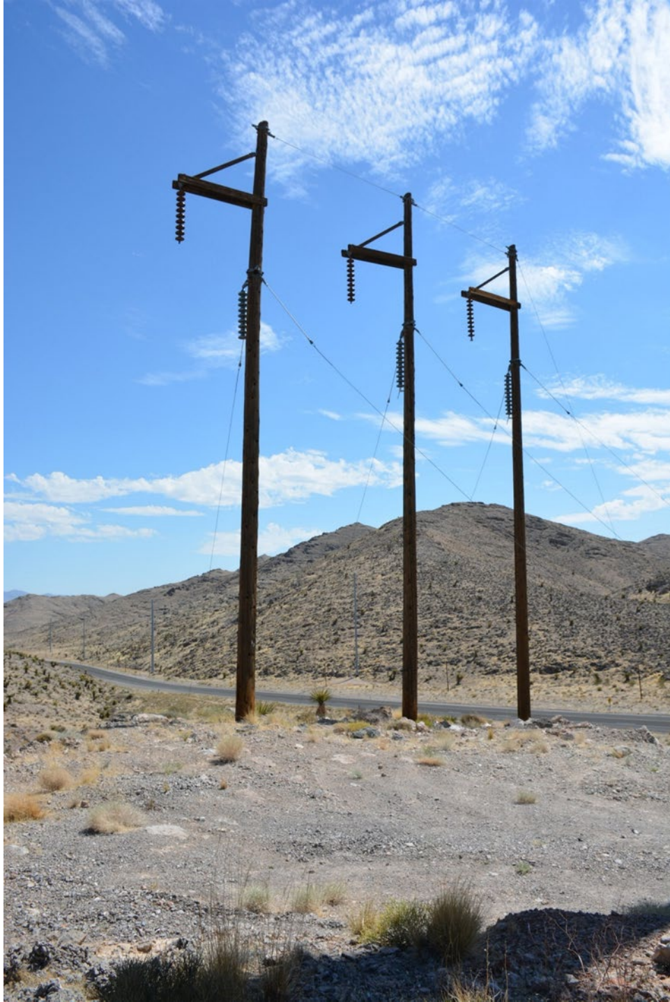
Photo No. 20. Dead end structure, facing east-northeast.
