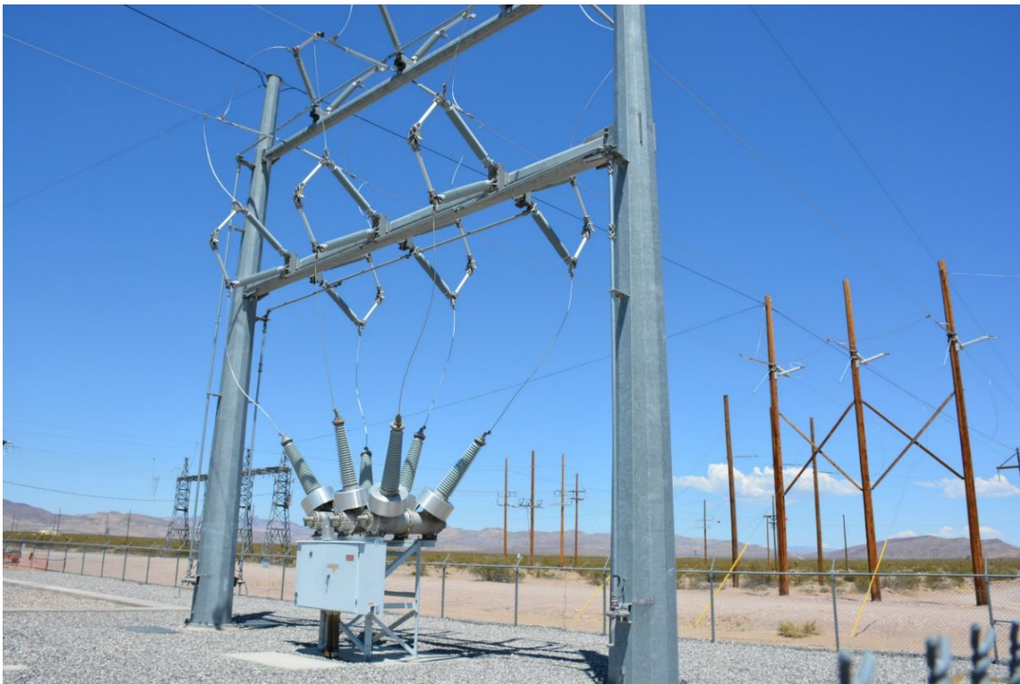
Photo No. 8. Frenchman Flat Substation 138 kV gas circuit breaker and incoming transmission line scaffolding, facing northwest.
