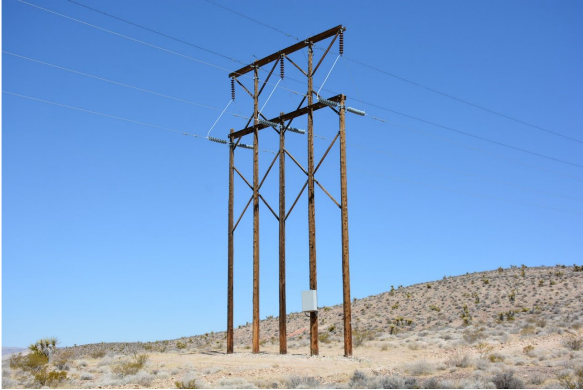
Photo No. 23. High tension suspension structure, oblique view, facing west-northwest.
