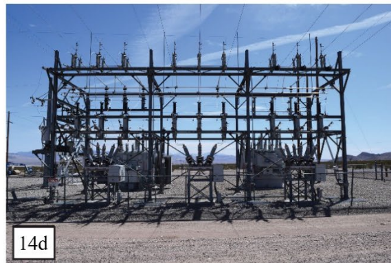
Figure 14a. Frenchman Flat Substation overview, facing west (2113MIT-C_006); Figure 14b. Detail of Frenchman Flat Substation 138 kV transformers (2113MIT-C_0011); Figure 14c. Detail of Frenchman Flat Substation 138 kV gas circuit breaker (2113MIT-C_0009); Figure 14d: Detail of Frenchman Flat Substation 34.5 kV distribution line system (2113MIT-C_0016).
