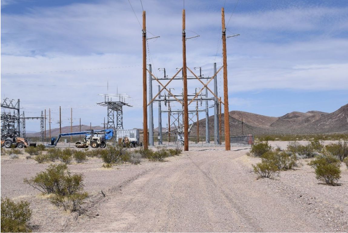
Figure 9. Typical three-pole dead-end structure (2113MIT-C_0004).
