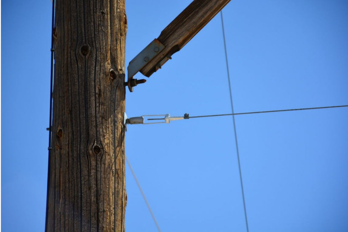
Photo No. 16. H-frame structure, detail of X-brace and pole tensioner hardware, facing north-northeast.
