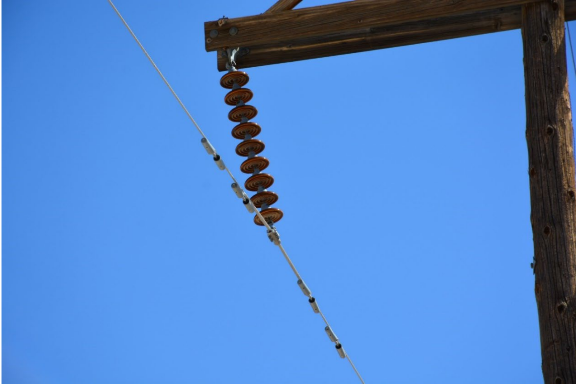
Photo No. 14. H-frame structure, detail of conductor wire and long-rod insulator attached to end of crossbeam, facing north-northeast.
