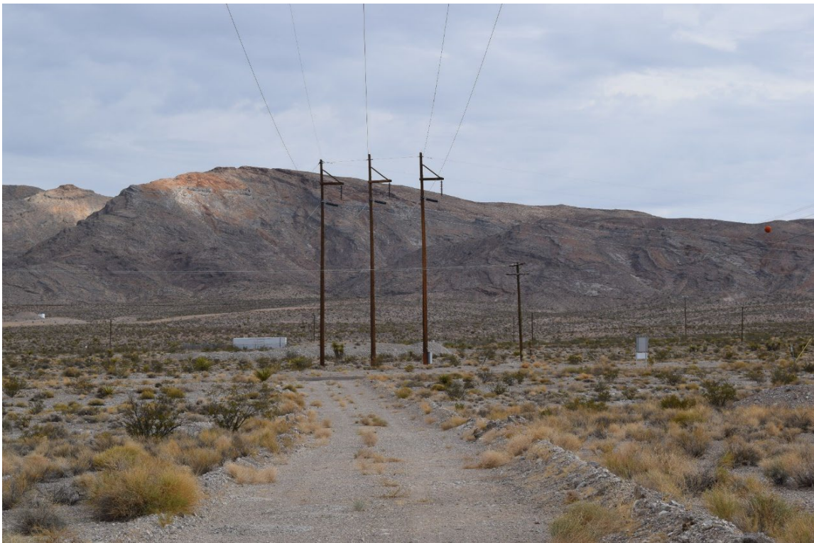
Photo No. 4. Dead end structure at turn in powerline, west side of Mercury, facing north-northwest (Mile 0.55).
