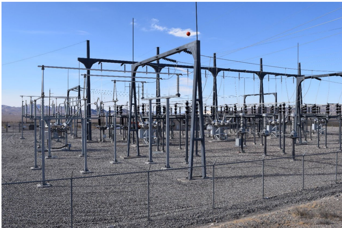
Photo No. 4. Mercury Switching Station, detail of lower bus system for NNSS 138 kV power transmission system, facing southwest (note scaffolding tower in mid-frame).
