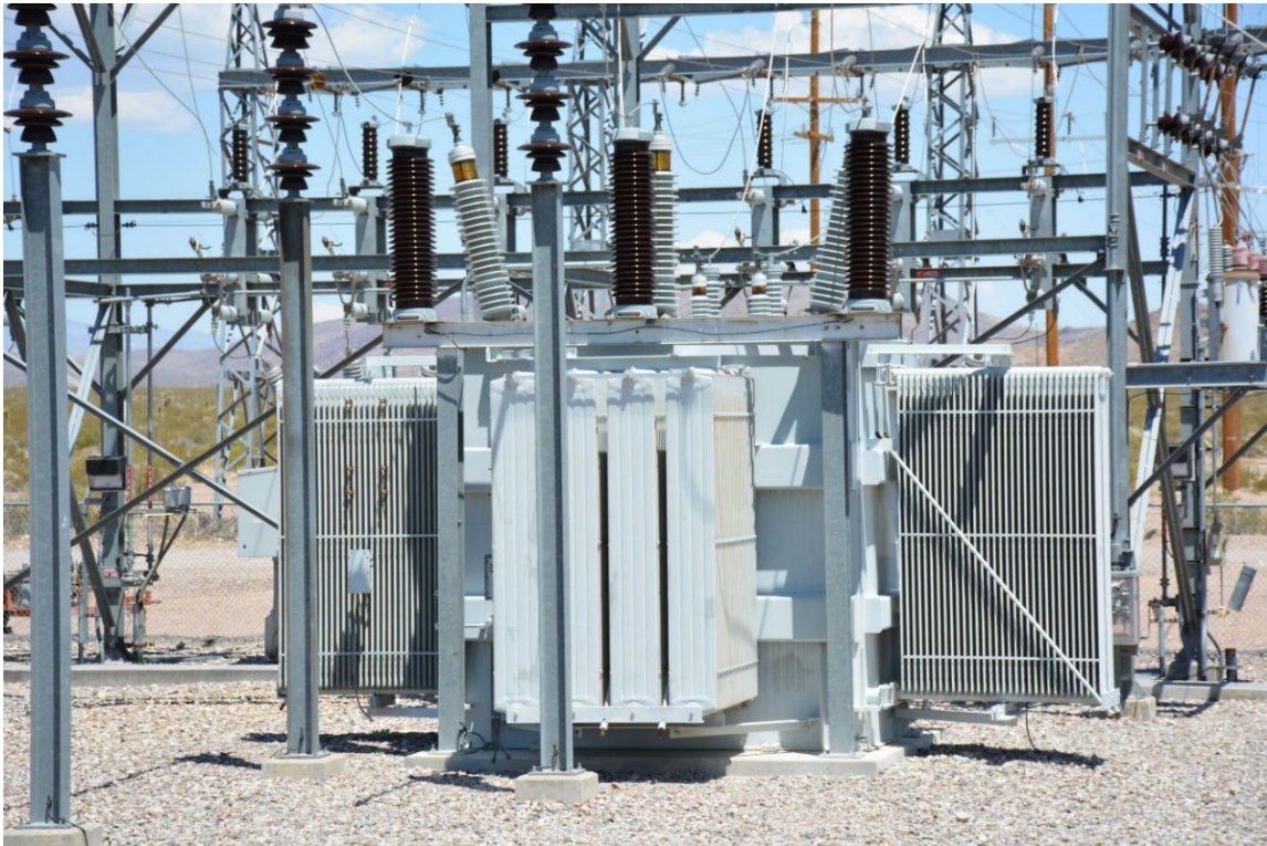
Photo No. 10. Frenchman Flat Substation, detail of old transformer model with cooling fins, facing north.
