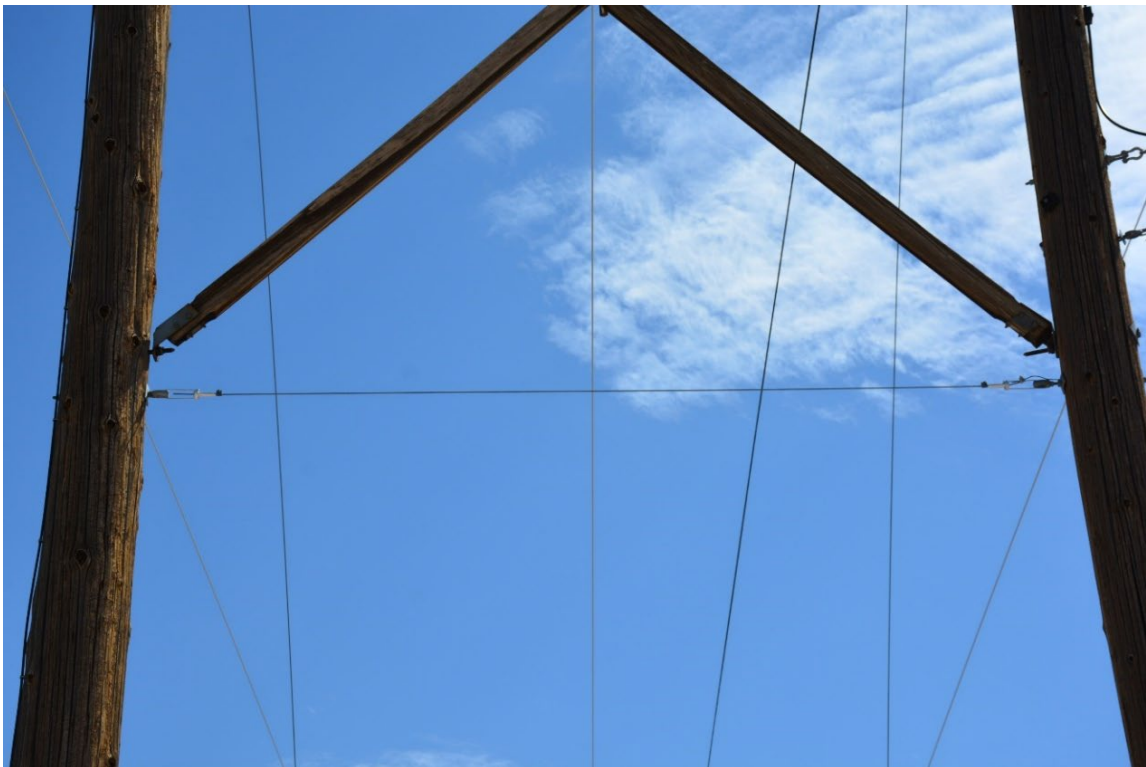
Photo No. 15. H-frame structure, detail of X-brace and pole tensioner, facing north-northeast.
