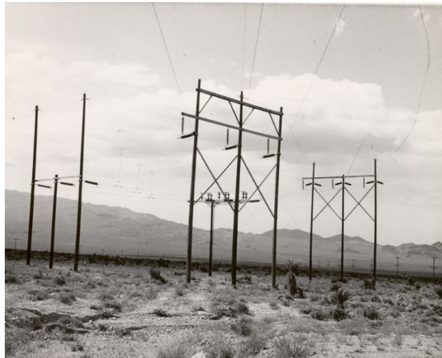
Figure 4. Series of dead-end structures near Mercury Switching Station, ca. 1958 (REEC0 1982:367-5).
