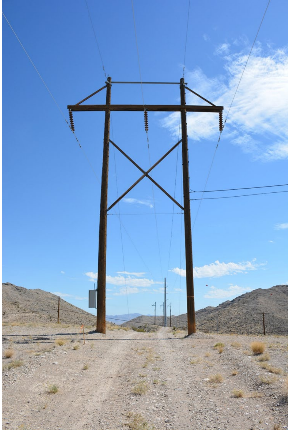
Photo No. 13. Typical H-frame structure with X-brace, facing north-northeast.
