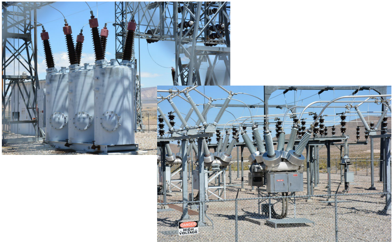
Figure 7. Detail of oil circuit breakers (left) and gas circuit breakers (right) (2113MIT-A_3107; 2113MIT-A_3012).
