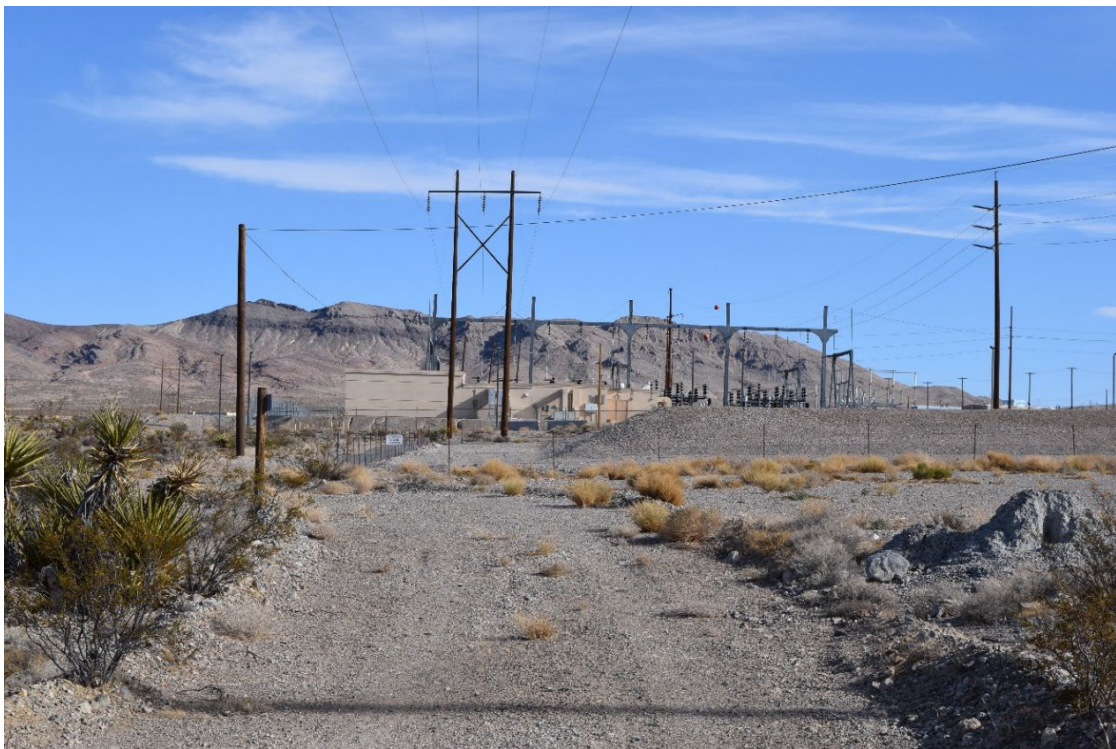
Photo No. 2. Mercury Switching Station, NV Energy 138 kV power transmission line junction with switching station, facing north (power line junctions with switching station on large scaffolding tower mid-frame; control houses are below and left of tower).
