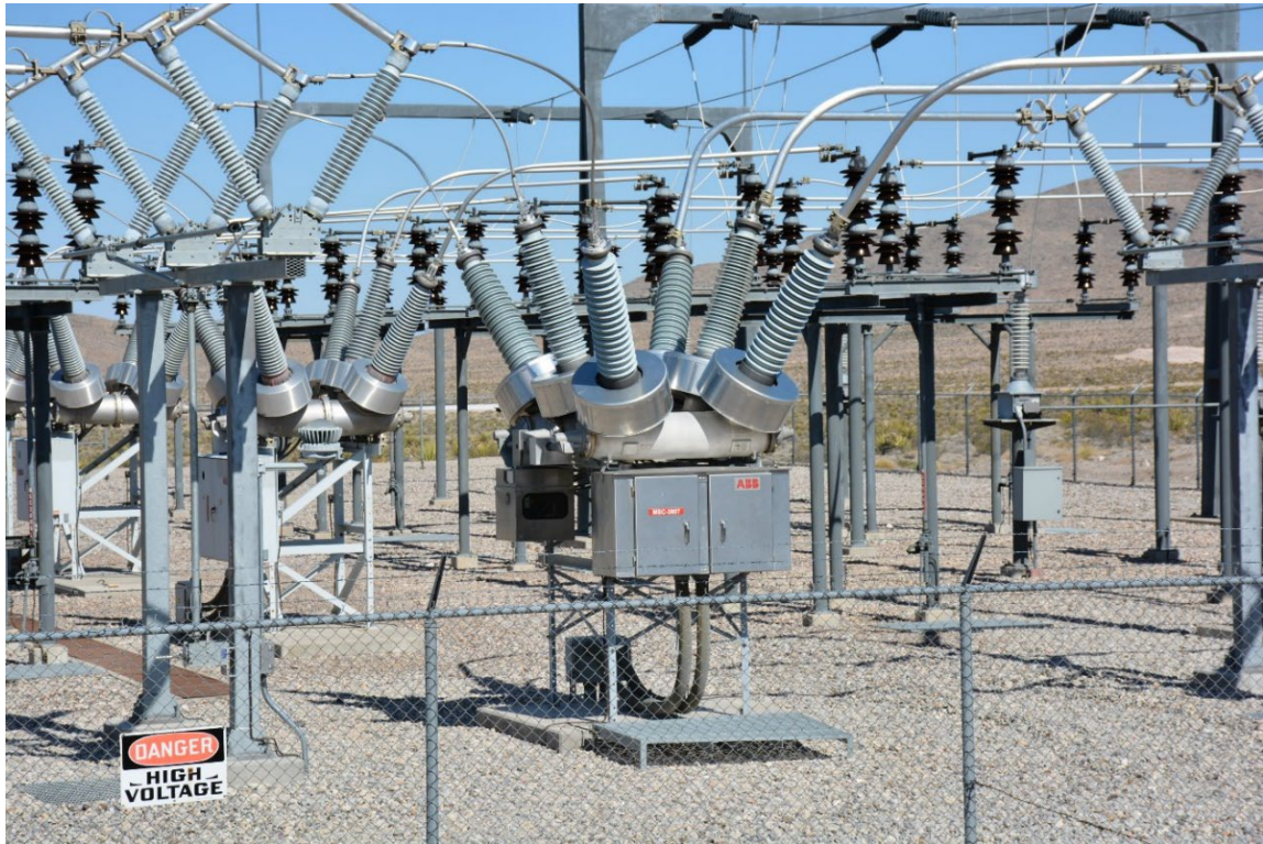
Photo No. 5. Mercury Switching Station, detail of gas circuit breakers, facing west-northwest.
