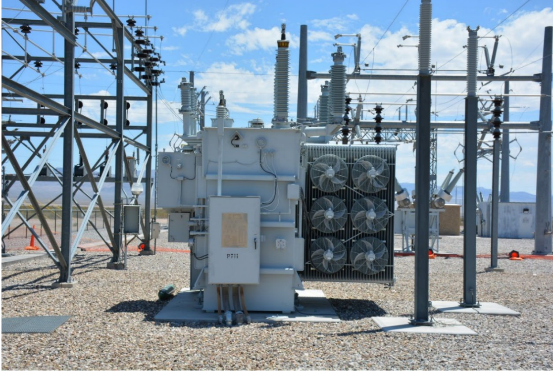
Photo No. 11. Frenchman Flat Substation, detail of new transformer model with cooling turbines, facing east.
