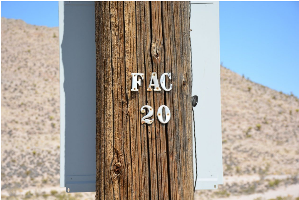
Photo No. 17. Detail of structure alphanumeric designation with ground wire on right and modern fiber optic box on opposite side, facing northwest.
