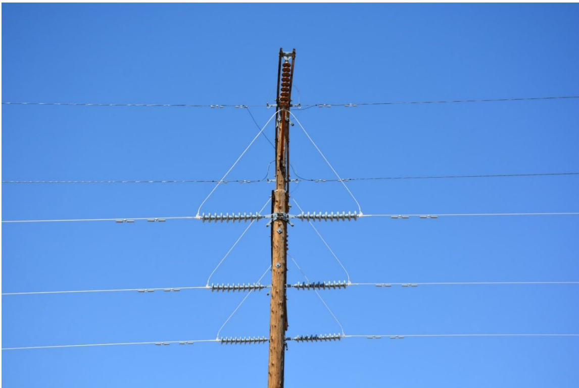
Photo No. 26. High tension suspension structure, detail of conductor wires, long-rod insulators, and associated hardware, facing west.
