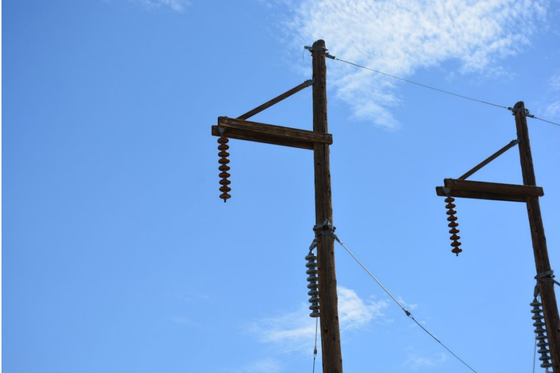
Photo No. 21. Dead end structure, detail of conductor wires, long-rod insulators, and hardware, facing east-northeast (lower insulator held transverse conductor wire, whereas upper insulator held angled conductor wire).
