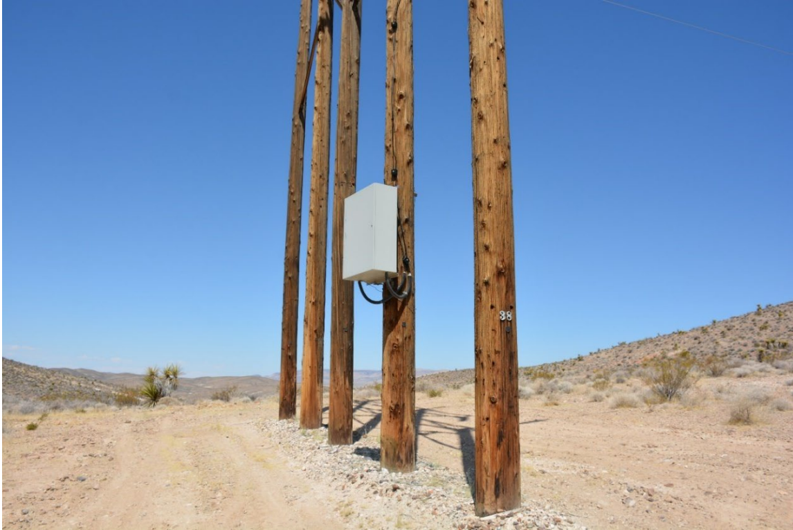
Photo No. 27. High tension suspension structure, detail of base with modern fiber optic box, facing west.
