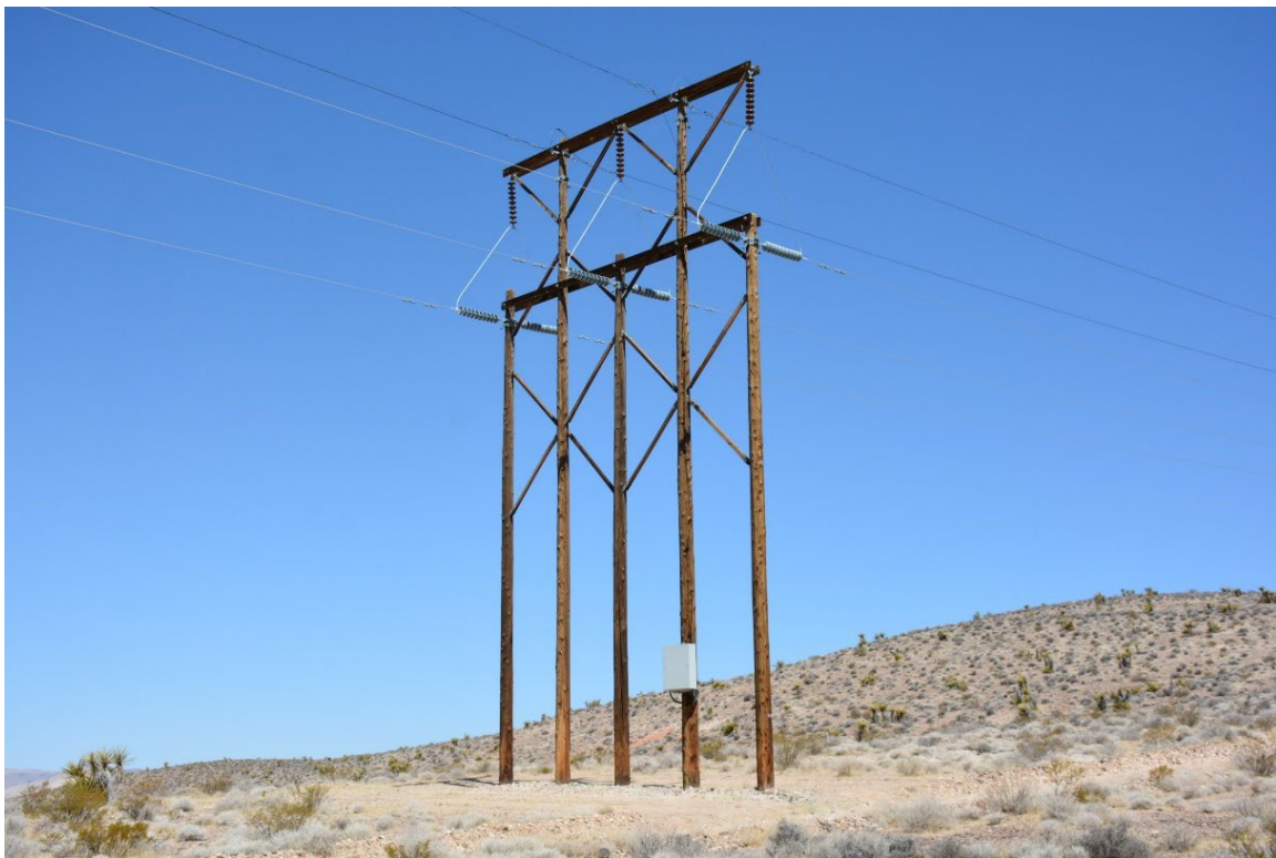
Figure 10. Typical five-pole high-tension suspension structure (2113MIT-A_3049).
