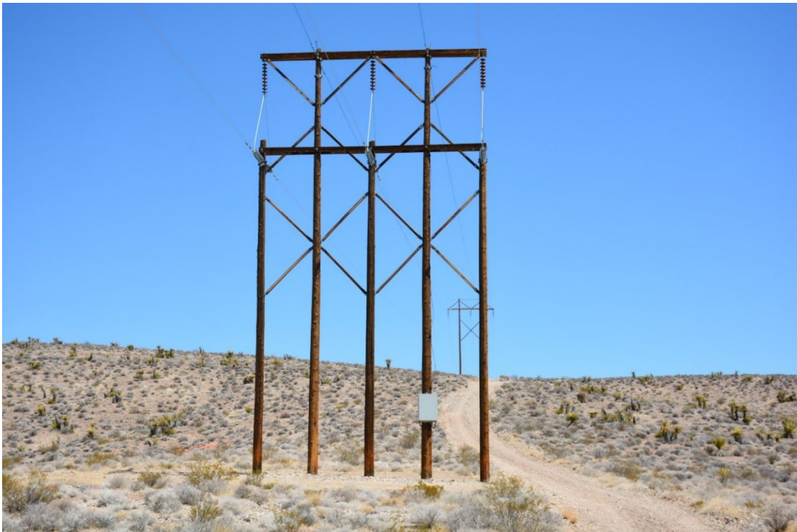
Photo No. 22. High tension suspension structure, frontal view, facing north.
