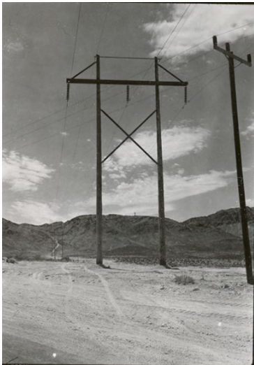
Figure 3. NNSS H-frame structure, ca 1963 (REEC0 1982:1673-11).
