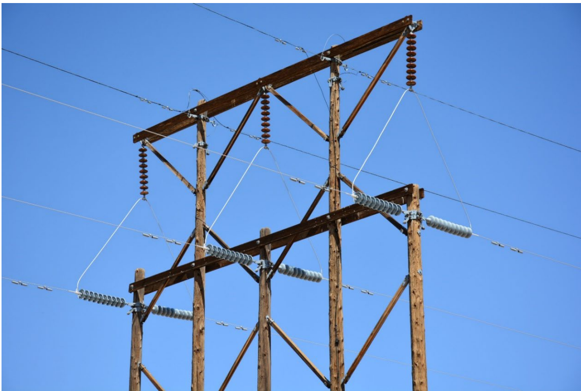
Photo No. 24. High tension suspension structure, detail with upper braces and power transmission hardware, facing west-northwest.
