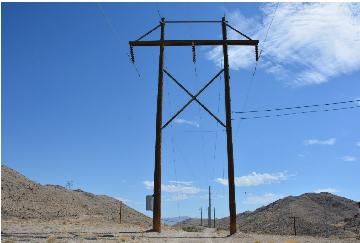
Figure 8. Typical H-frame structure (2113MIT-A_3020).
