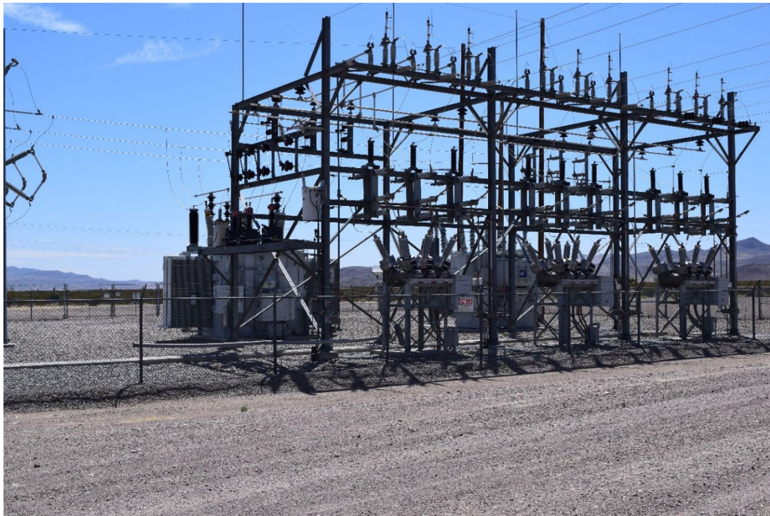
Photo No. 12. Frenchman Flat Substation 34.5 kV distribution system scaffolding and circuitry, facing southwest (transformers in background, scaffolding and 34.5 kV electrical circuitry foreground, 34.5 kV gas circuit breakers below scaffolding and circuitry).
