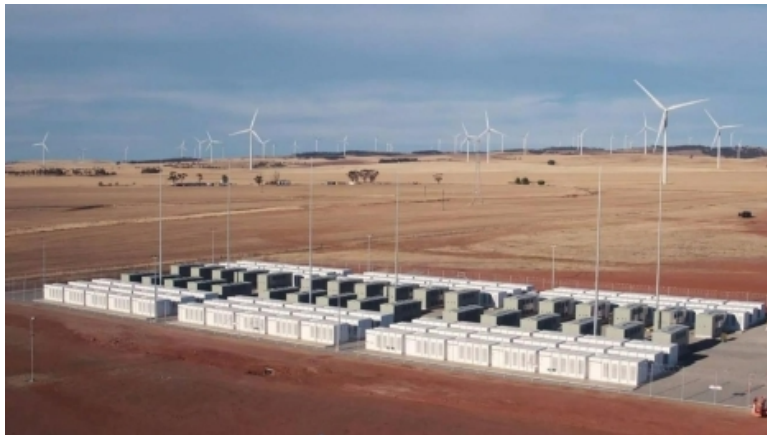
Tesla 100 MW / 129 MWh ESS Australia - Grid stability
