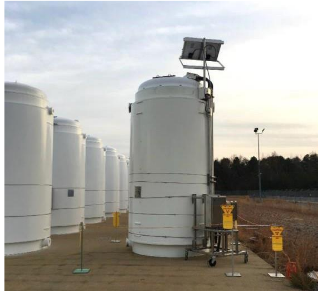
Loaded TN-32 for the High Burnup Demo at North Anna NPP. The solar panel is powering the 63 thermocouples inside the canister. Photo Credit: North Anna NPP
