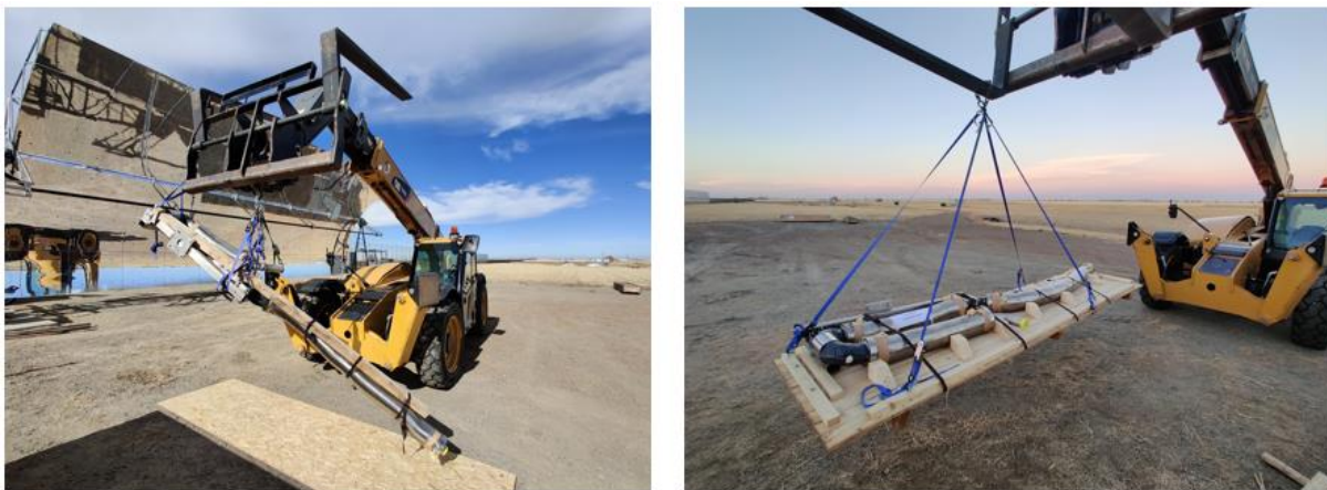
Figure 29. Flex hose rigging and lifting
