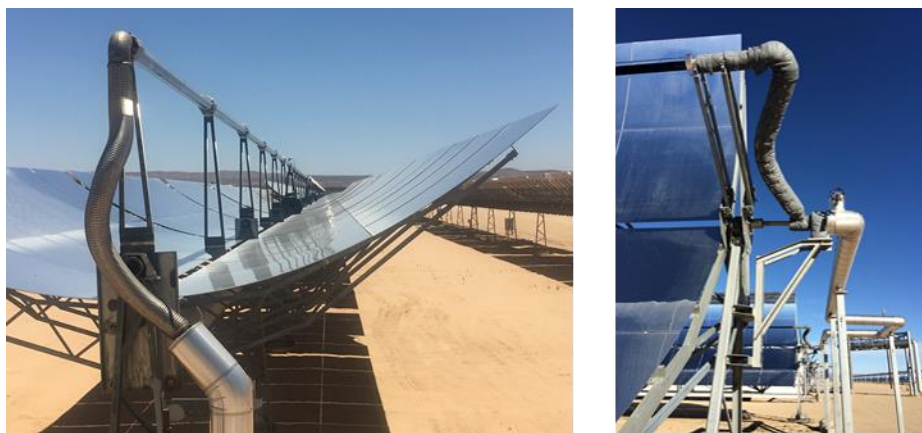
Figure 2. LS-2 Flex Hose at SEGS III (left) and flex hose assembly with rotary joint at Mojave Solar Project (right)
