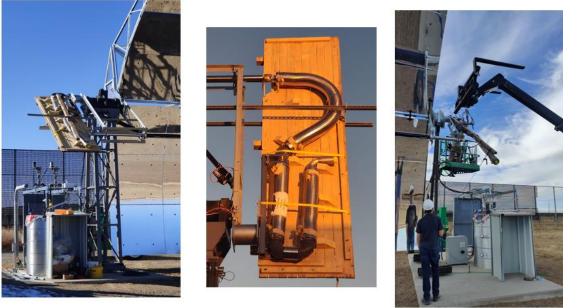
Figure 30. Flex hose placement and staging for welding
