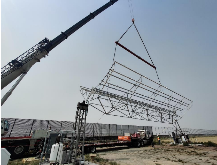
Figure 26. Crane Operation to Relocate SunBeam™ Module
