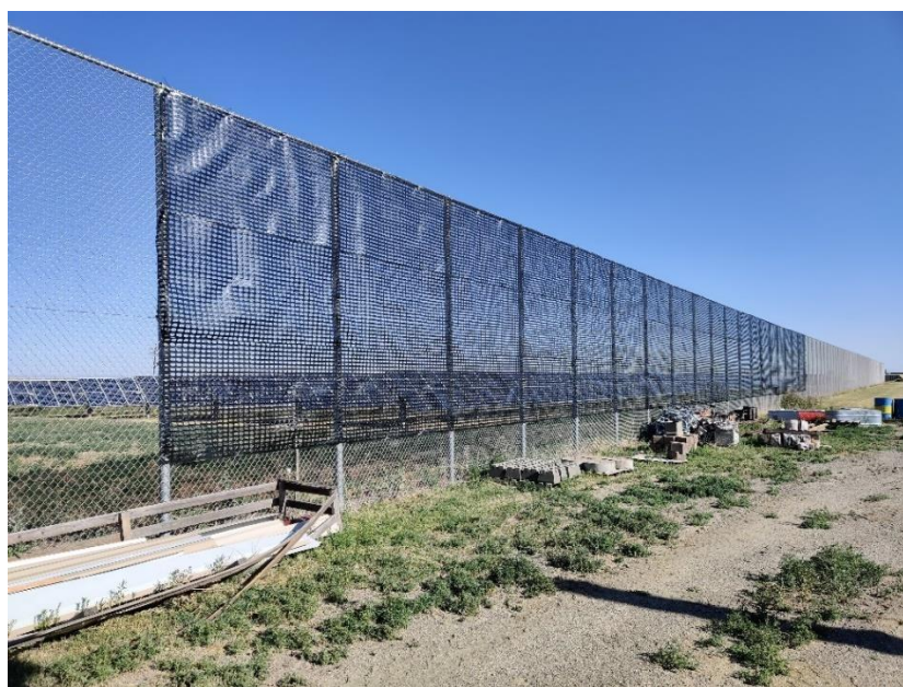
Figure 25. Wind Fence Installation on Existing Fence
