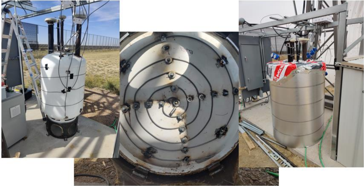
Figure 28. Salt Tanks Heat Trace & Insulation
