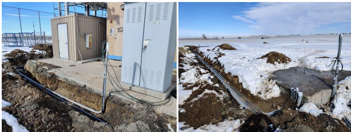
Figure 20. Picture of Underground Conduit Installed in Q1 2020
