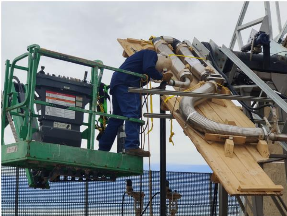
Figure 31. Flex hose placement and welding
