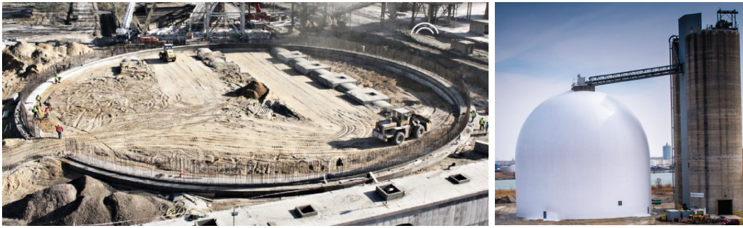
Figure 10. Monolithic concrete dome storage vessels. (Left) foundation construction of a large concrete dome with discharge tunnel. (Right) Dome with charging chute. Images are property of Dome Technology and are used with permission.
