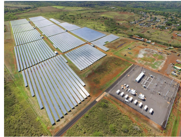
Saft 6 MW / 4.2 MWh ESS Kauai - Grid Stability
