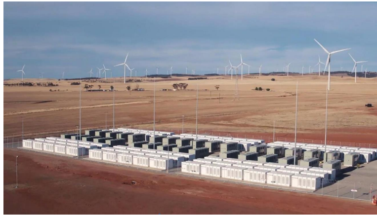
Tesla 100 MW / 129 MWh ESS Australia - Grid stability
