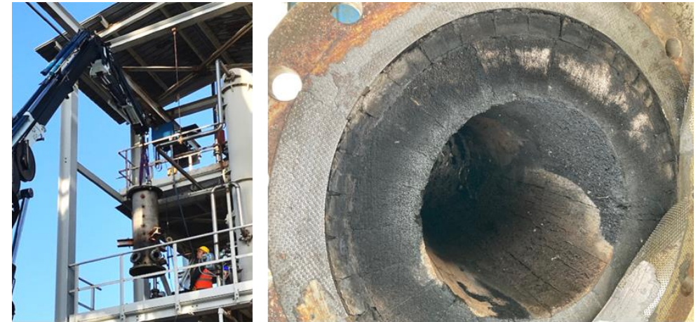
Reactor removal and refractory layer before the reconstruction
