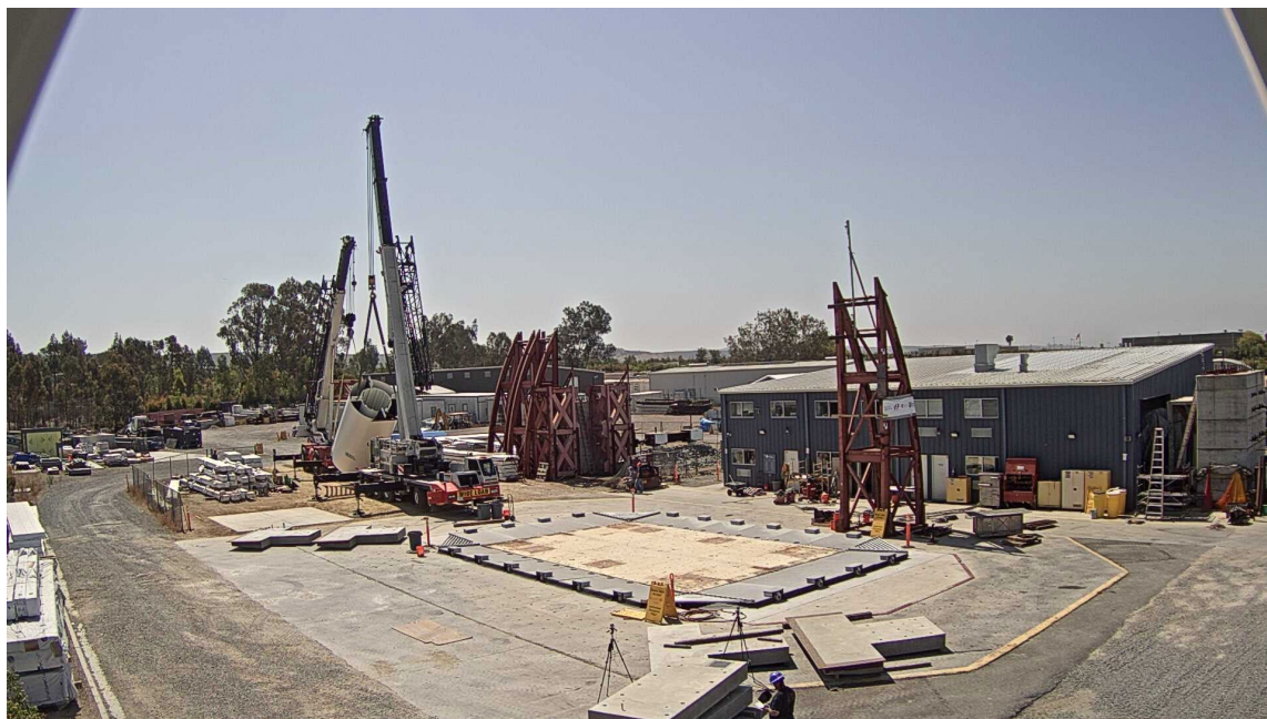
Figure 3-17. Cask Unloading at the Shake Table Facility at the UCSD.
