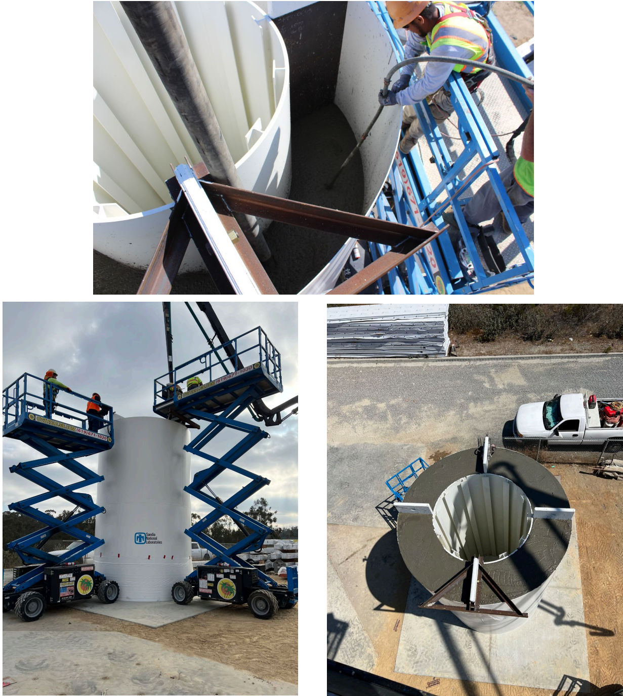
Figure 3-18. Pouring Concrete into the Cask (top and bottom left) and Filled with Concrete Cask (bottom right).
