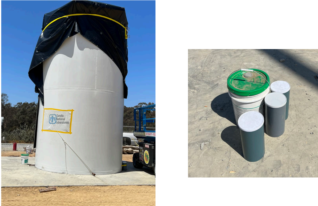
Figure 3-19. Completed Vertical Cask Covered with the Tarp (left) and Concrete Samples (right).
