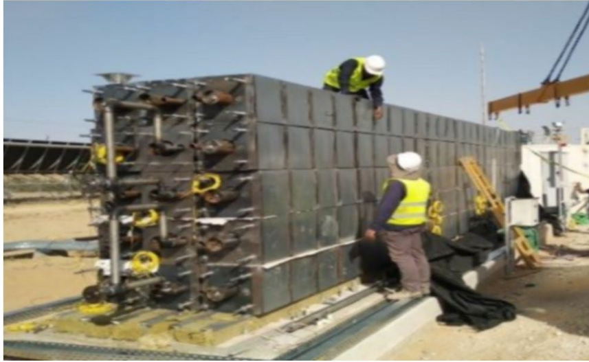
Figure 6-3. Photo of a Brennmiller Energy bGen TM thermal storage module internals (bCubes)
