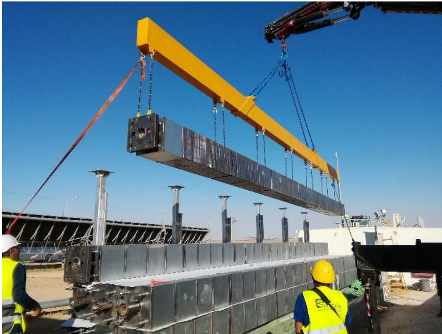
Figure 2-3. Photo of a Brenmiller Energy bGen TM thermal storage module internals (bCubes)
