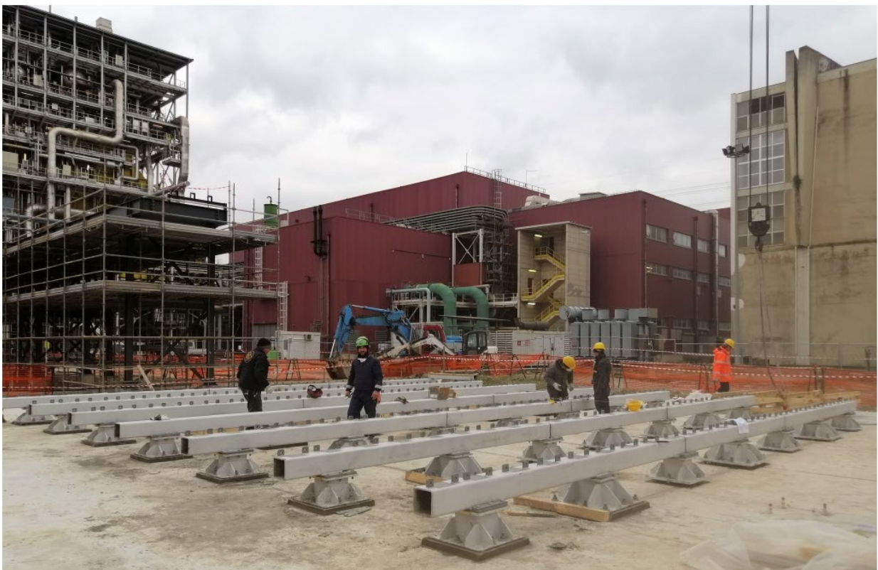
Figure 4-6. Construction of Foundation for Stacking Arrangement
