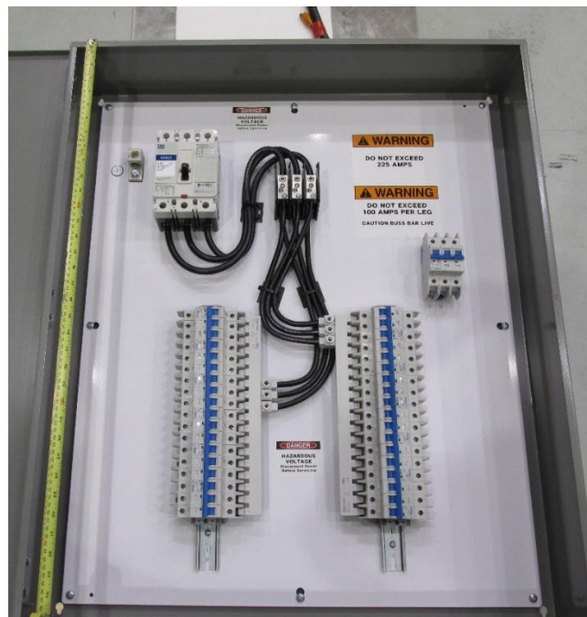
Figure 2-2. Circuit breakers installed in breaker panel
