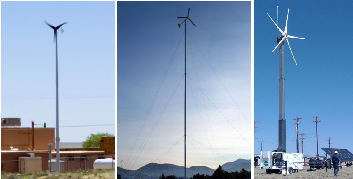
Figure 6. Single-piece, monopole tower (left, Pika Energy turbine, NREL PIX 31470), segmented, guyed tower (center, Bergey Windpower turbine, NREL PIX 16742), and telescoping tower (Uprise Energy turbine, Idaho National Lab)
