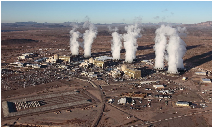
FIGURE 1: Aerial photograph of the Palo Verde Generating Station.
