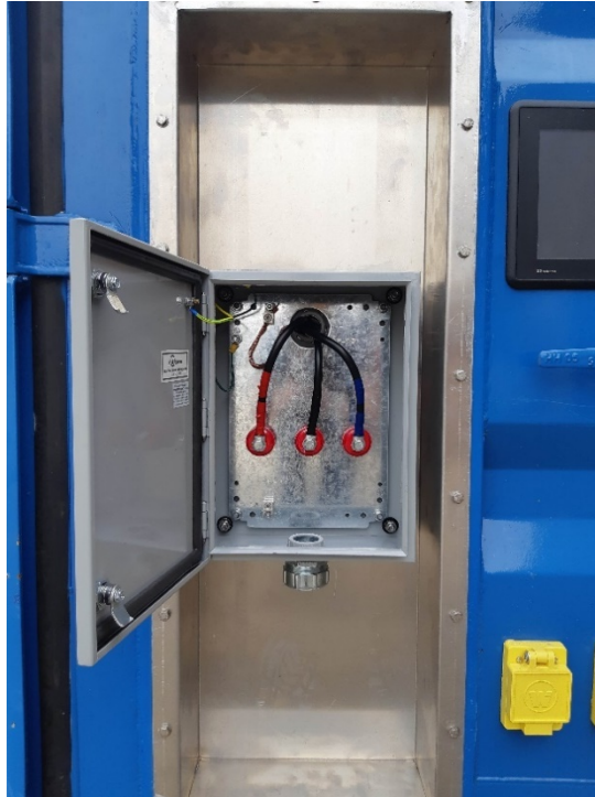
Figure 3: New recessed connector panel/box mounted on the MarFC unit.
