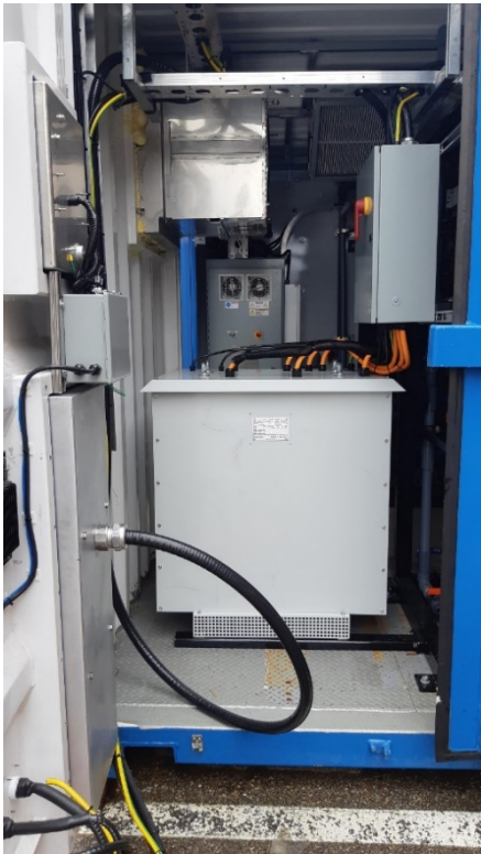
Figure 1: New transformer installed
