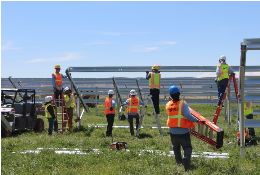
Interns, Grid Employees and Volunteers during construction
