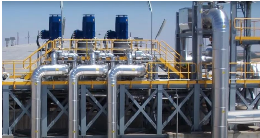
Figure 33. Molten salt pumps (Flowserve.com).
