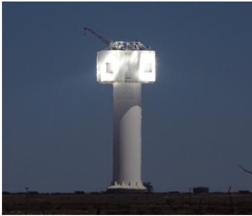
Figure 29. Left: Multi-cavity molten-salt receiver at Khi Solar One . Right: Particles falling over catch-and-release troughs in a cavity receiver during testing at Sandia.
