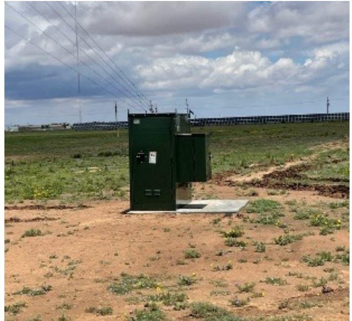
New switchgear with enhanced safety features to allow for safe switching to support experiments where SWiFT turbines are providing power to the TTU GLEAMM microgrid. Image credit: Brandon Davis
